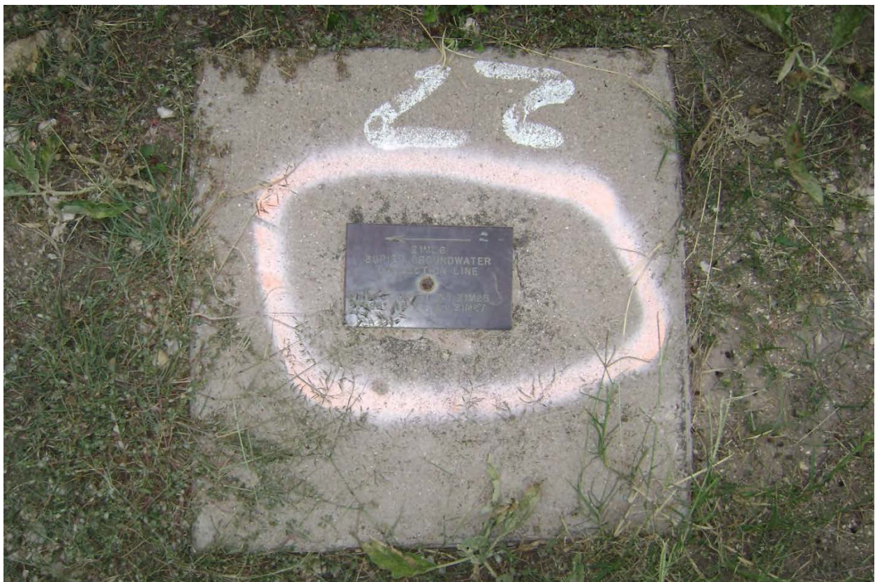
Site Photograph A-8 Groundwater collection line marker near proposed levee station 24+00
