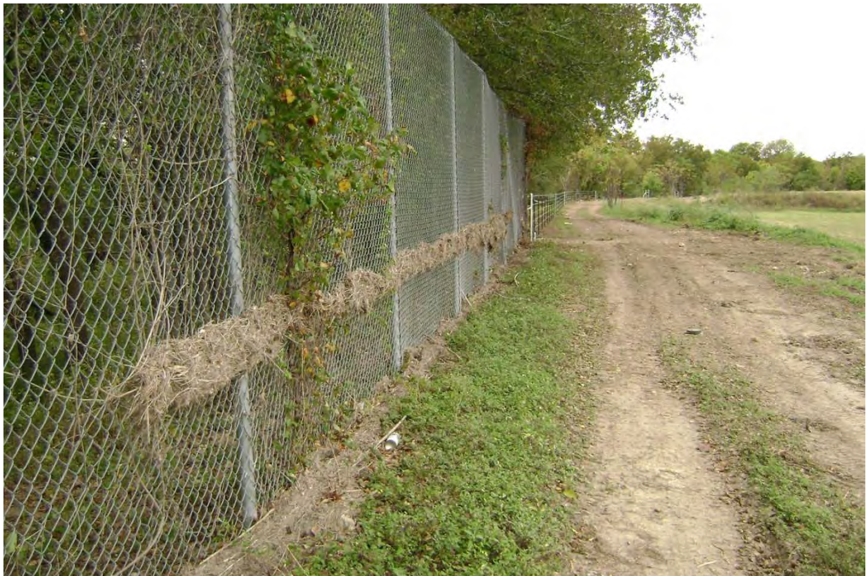
Site Photograph A-6 High water mark on perimeter fence from May 2013 flooding along Leon Creek near proposed levee station 19+50
