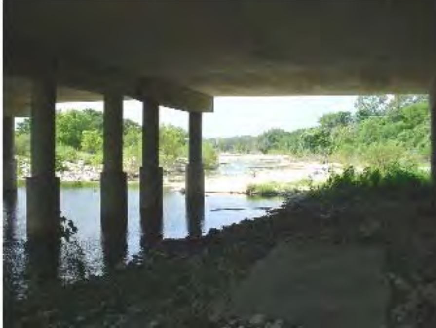
Leon Creek - Culebra St Bridge Piers Looking Downstream
