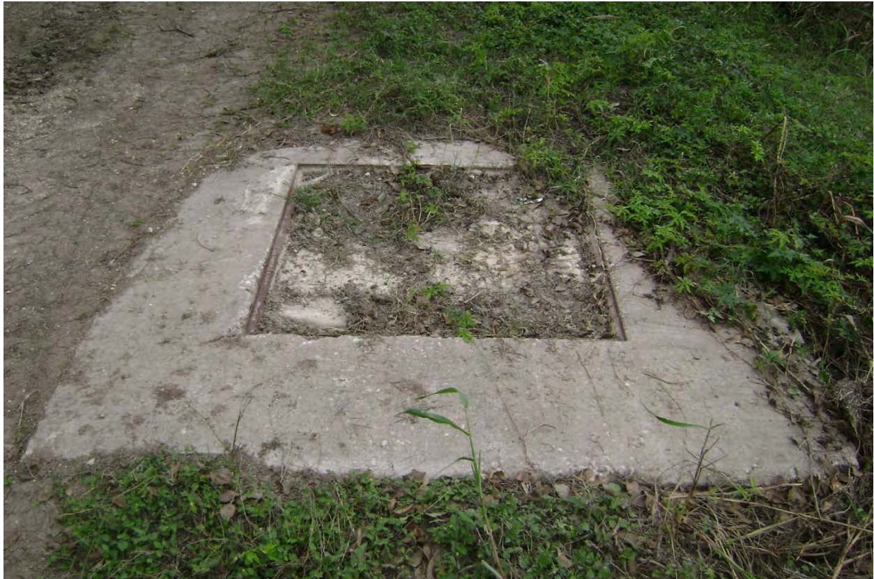
Site Photograph A-5 Plugged groundwater recovery well near proposed levee station 14+00
