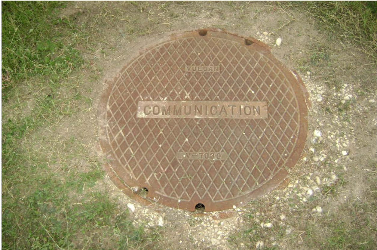
Site Photograph A-17 Communication manhole near proposed floodwall and water/gas line relocation area
