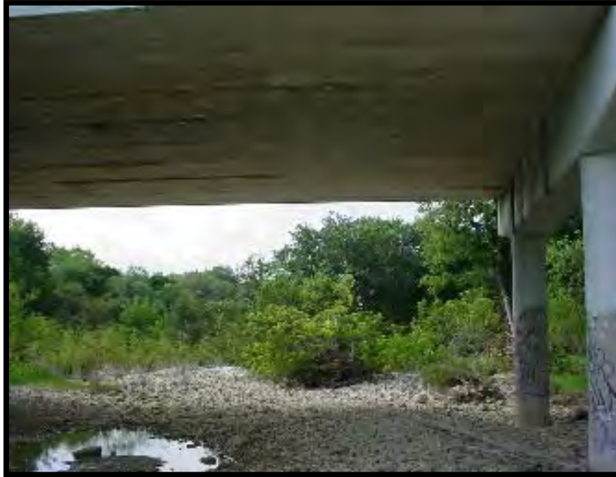
Leon Creek - Prude Rd From Under Bridge Looking Downstream
