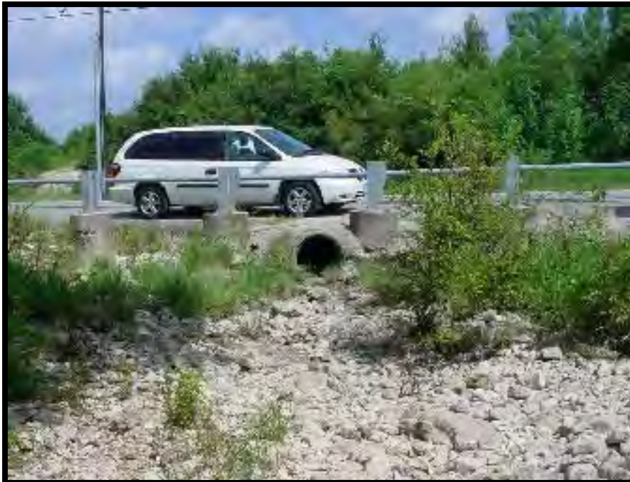
Culebra Creek - DS of Old Grissom Rd Culvert at Low Water Crossing
