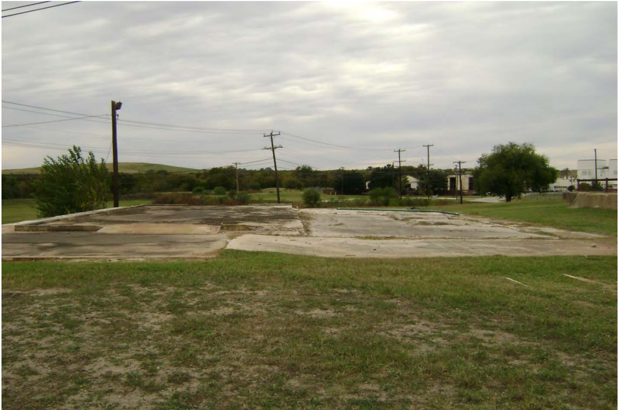
Site Photograph A-1 Concrete remaining from former Industrial Wastewater Treatment Plant to be removed for proposed levee access drive, gate, and patrol road at station 12+00
