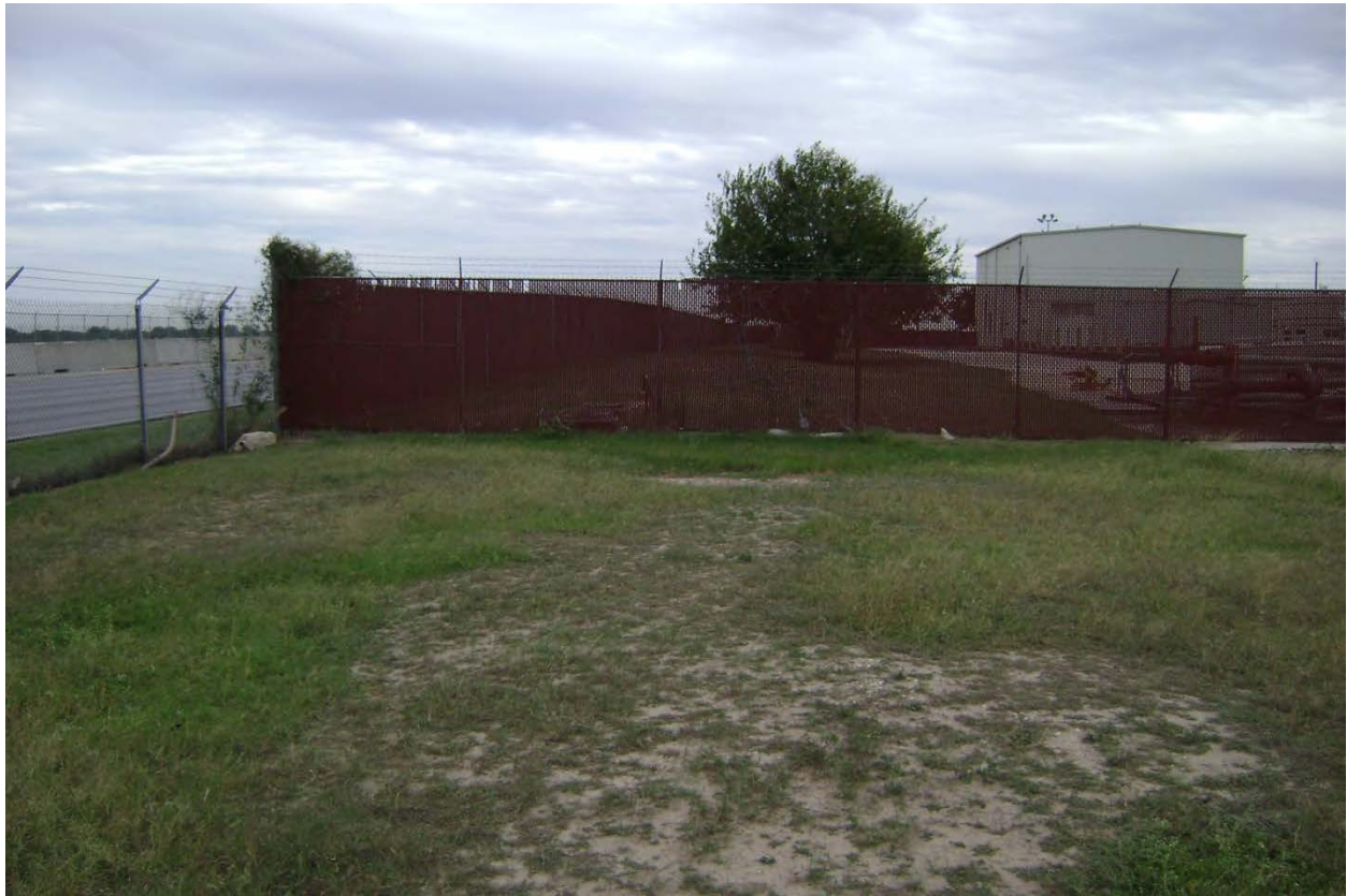
Site Photograph A-18 Property at end of proposed floodwall
