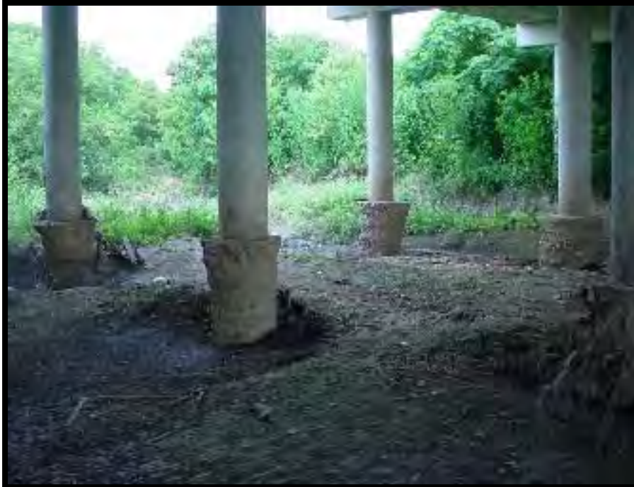
Culebra Creek - Culebra St Bridge Piers Scouring
