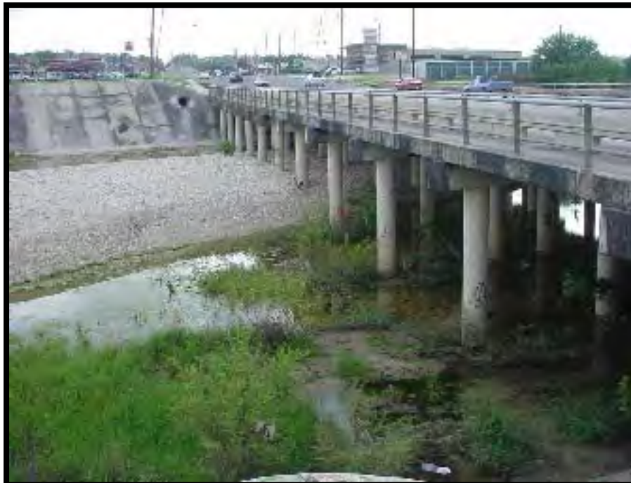
Leon Creek - Grissom Rd Bridge Looking Downstream from Upstream side
