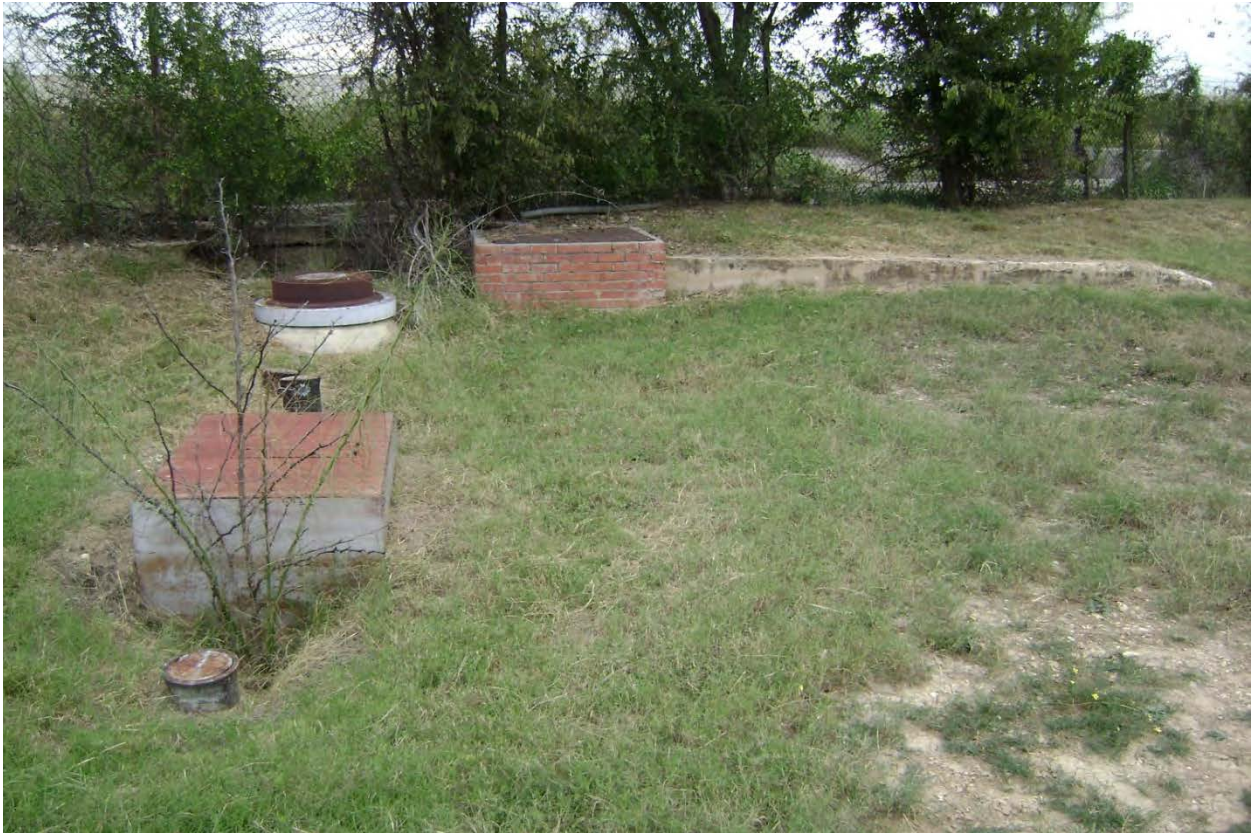
Site Photograph A-15 Existing water and gas valves along proposed floodwall
