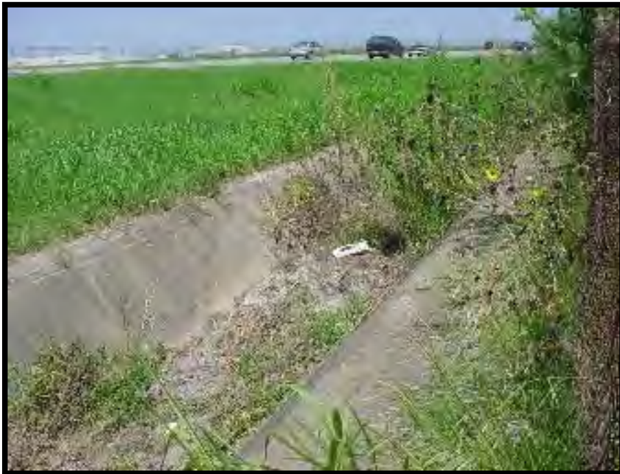
Leon Creek - PSA Test Cell Area SW Drainage Ditch
