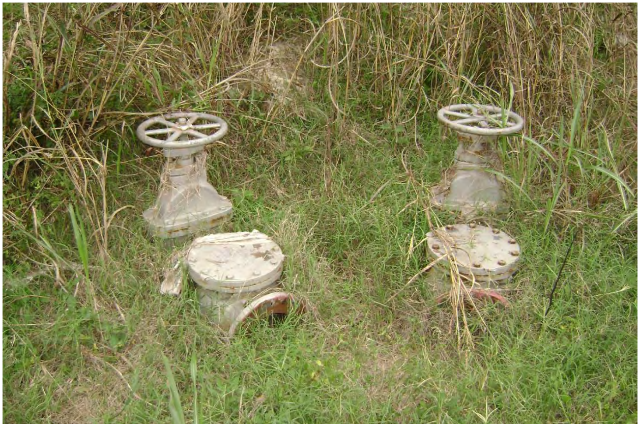
Site Photograph A-4 Valves along proposed levee side slope near station 15+30
