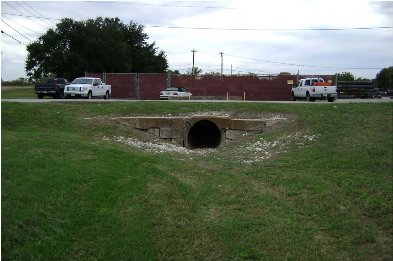
Site Photograph A-19 Reinforced concrete drainage pipe (48" diameter) to be outfalled into proposed sump
