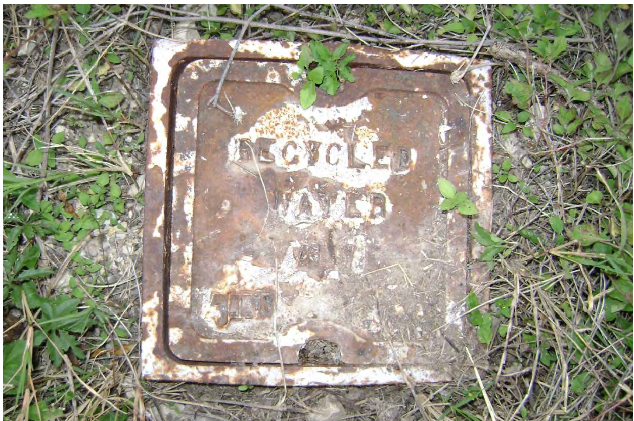
Site Photograph A-12 Close-up view of recycled water valve box along proposed levee side slope near station 28+60
