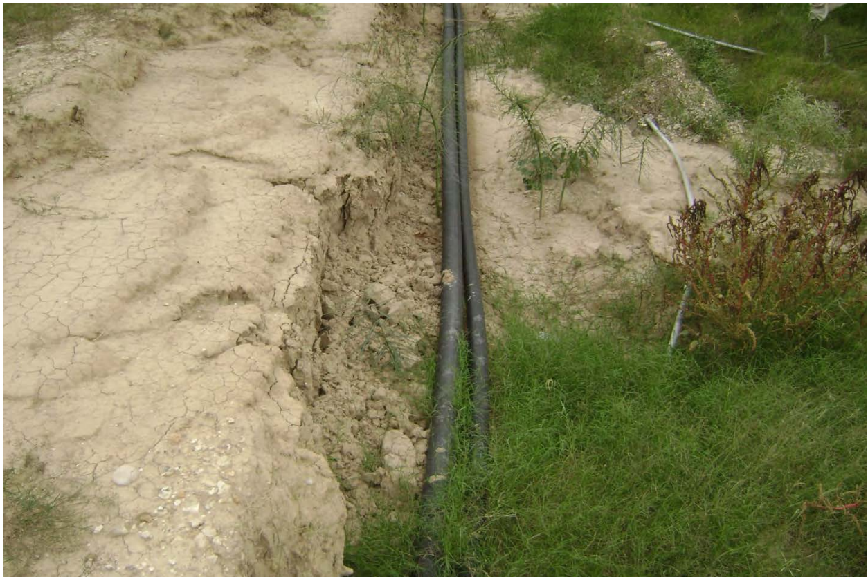
Photograph A-22 HDPE pipe and metal conduit for groundwater recovery system along existing flood control berm to be removed for proposed sump
