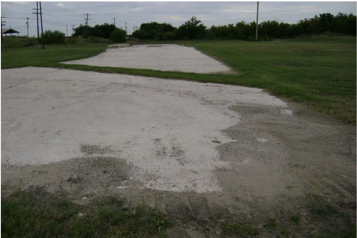
Site Photograph A-20 Concrete from former Industrial Wastewater Treatment Plant to be removed for proposed sump at former sludge drying beds/dewatering facility (IRP Site SD-2)
