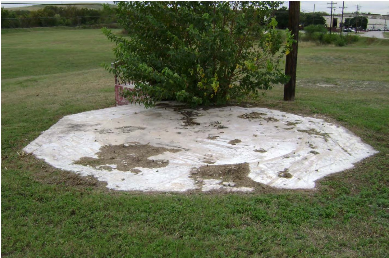
Site Photograph A-2 Concrete remaining from former Industrial Wastewater Treatment Plant to be removed for proposed levee side slope near station 12+60
