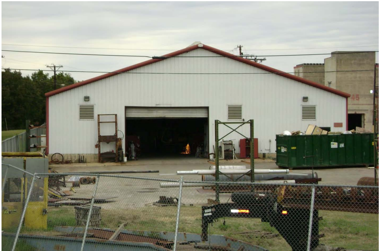
Site Photograph A-7 Metal Building along proposed levee side slope and surface drainage ditch near station 28+00
