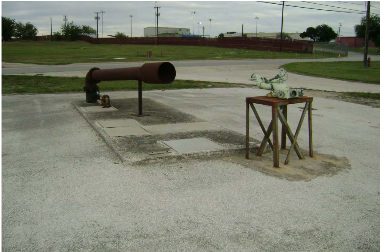
Photograph A-21 Concrete and structures to be removed for proposed sump
