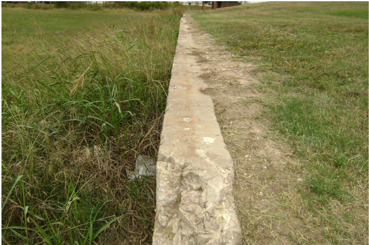
Site Photograph A-3 Concrete wall at former sludge dewatering basin near station 14+00
