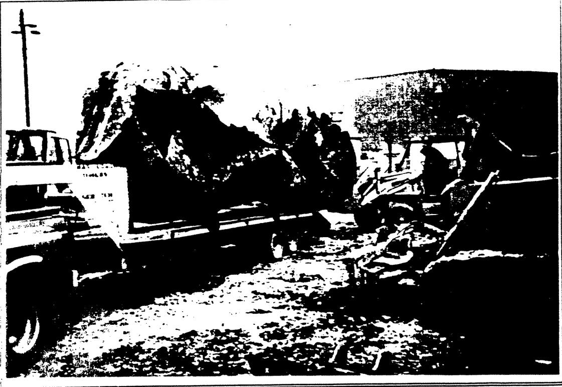
5. UST loaded and strapped for hauling to scrap metal recycling facility.
