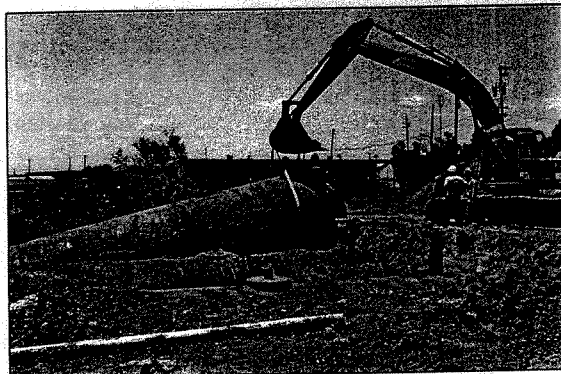
Underground Storage Tank Removals at the Fuel Farm.
