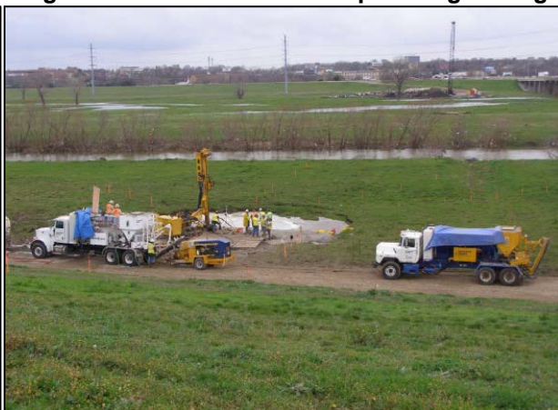
Figure 20 - Photo of the Remedial Grouting
