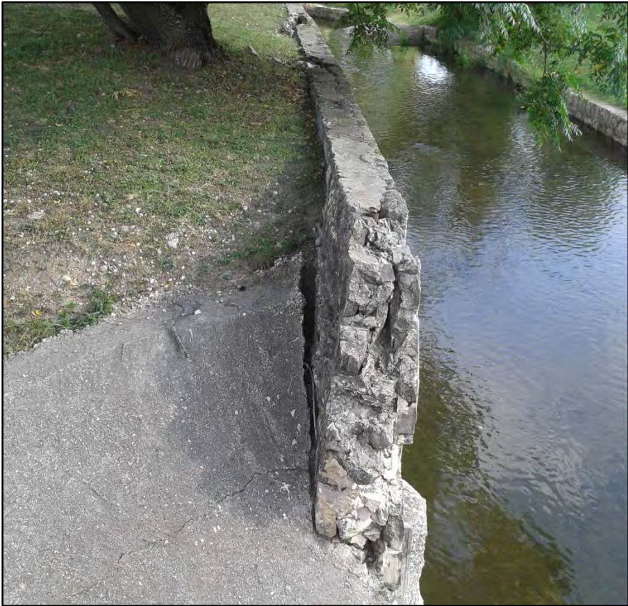
Figure 11. Separation of masonry wall from bank due to lack of proper anchoring.
