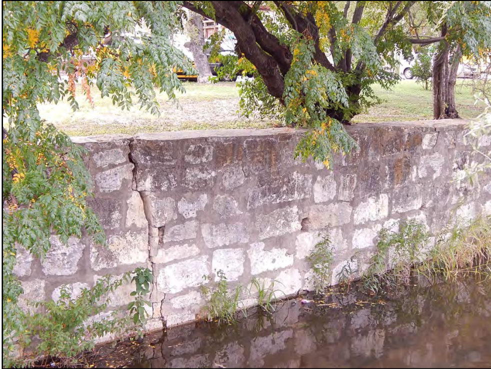
Figure 12. Extensive wall failure of stone masonry wall.
