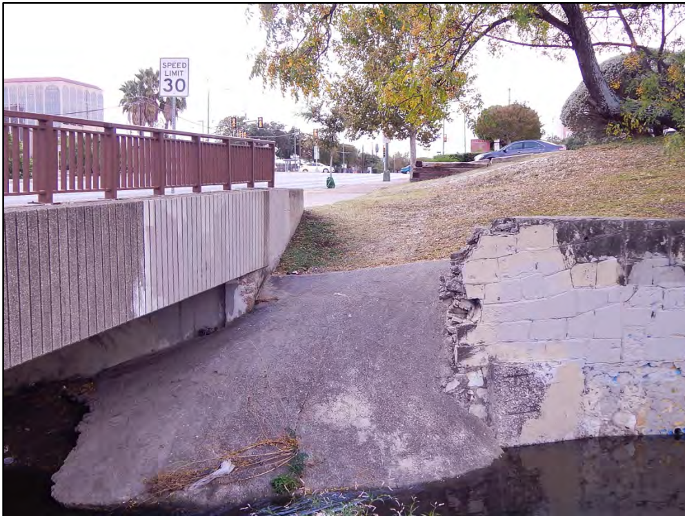
Figure 13. Bridge footing that damaged stone masonry wall at W. Travis St.
