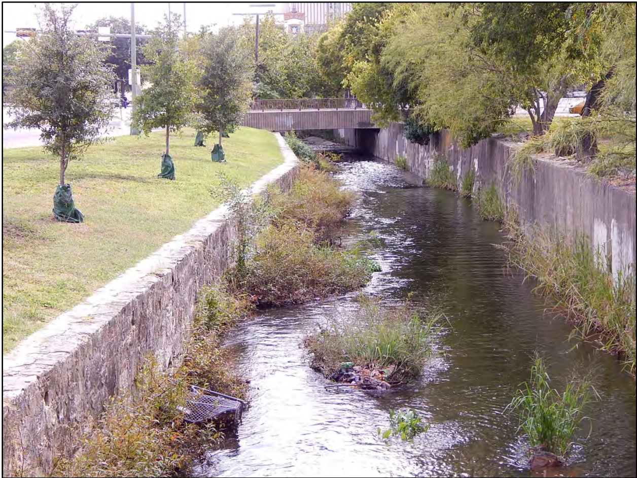
Figure 8. Upper reach of San Pedro Creek just north of Travis Street Bridge.
