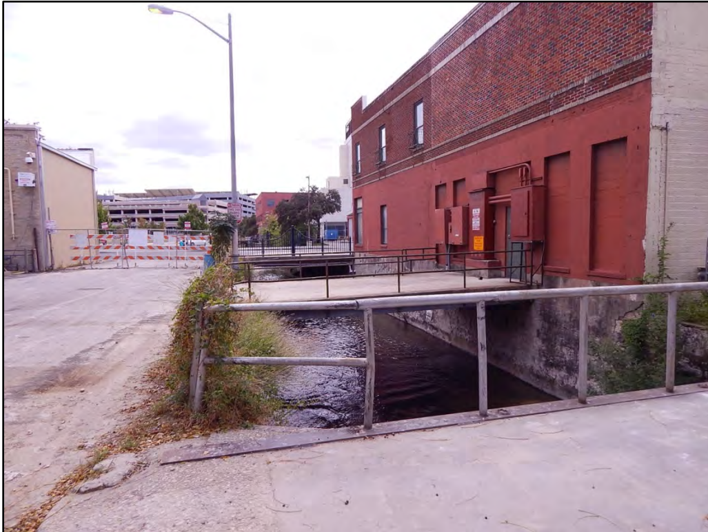
Figure 7. Small supply bridges in foreground near Dolorosa Street Bridge in background crossing San Pedro Creek.
