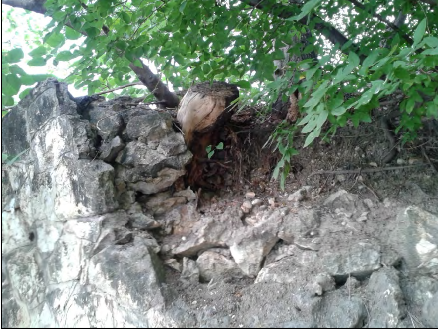
Figure 10. Stone masonry wall damage caused by roots.
