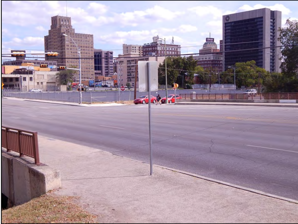
Figure 6. Multi-lane vehicular and pedestrian bridge at W. Martin Street.
