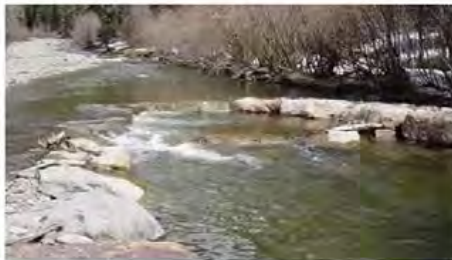
Cross vane structure with step on the East Fork Piedra River, CO
