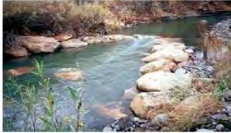
Cross vane installed on the lower Blanco River, CO
