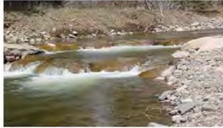
Cross vane/step-pool on the East Fork Piedra River, CO
