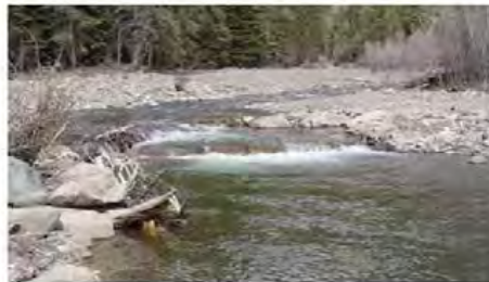
Cross vane/rootwad/log vane step-pool, converting a braided D4 → C4 stream type on the East Fork Piedra River, CO
