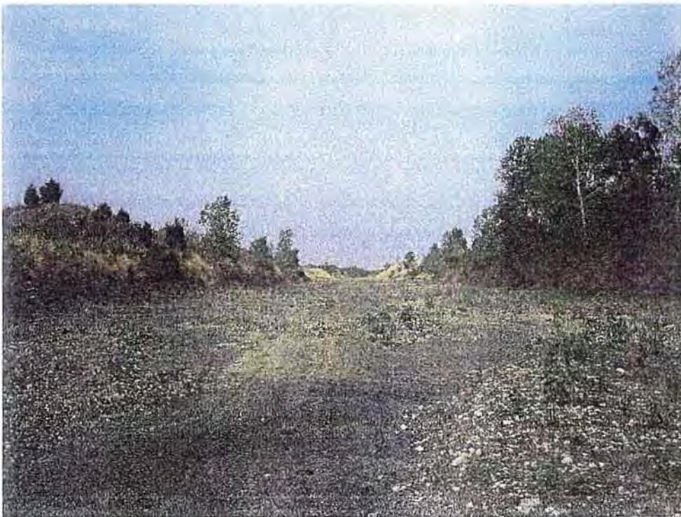
P2. 904 bridge looking east
