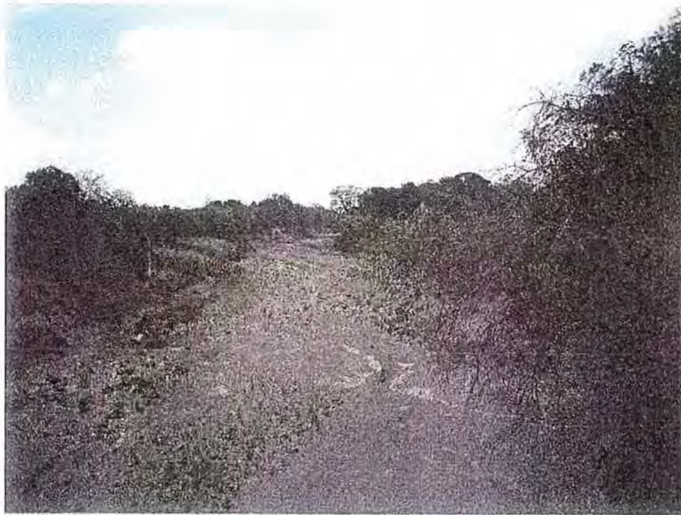
P3. 2920 bridge looking east
