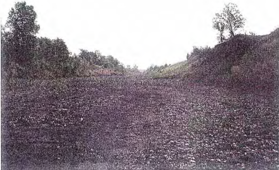
P1. 904 bridge looking west.
