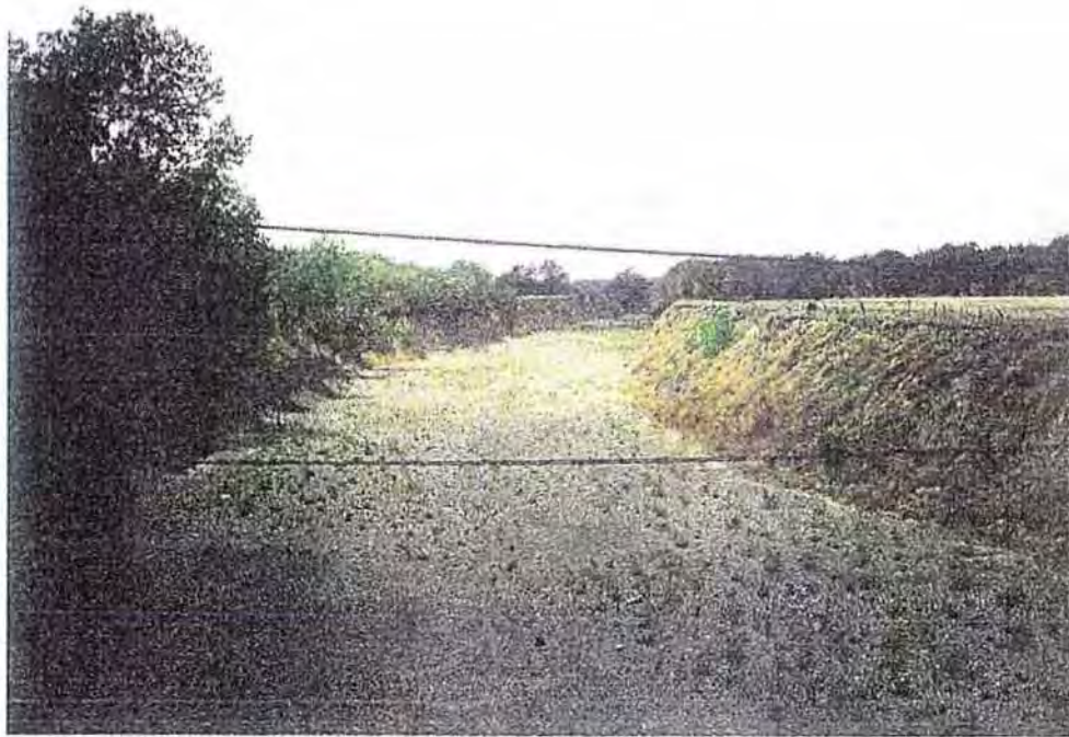
P4. 2920 bridge looking west
