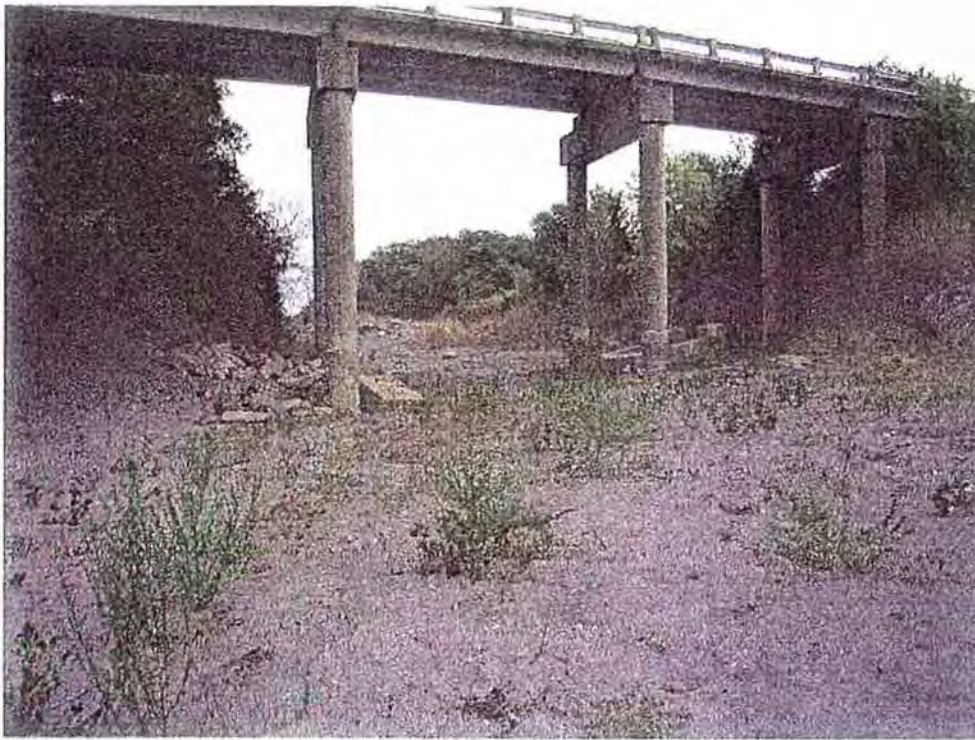
P5. 64 bridge looking east
