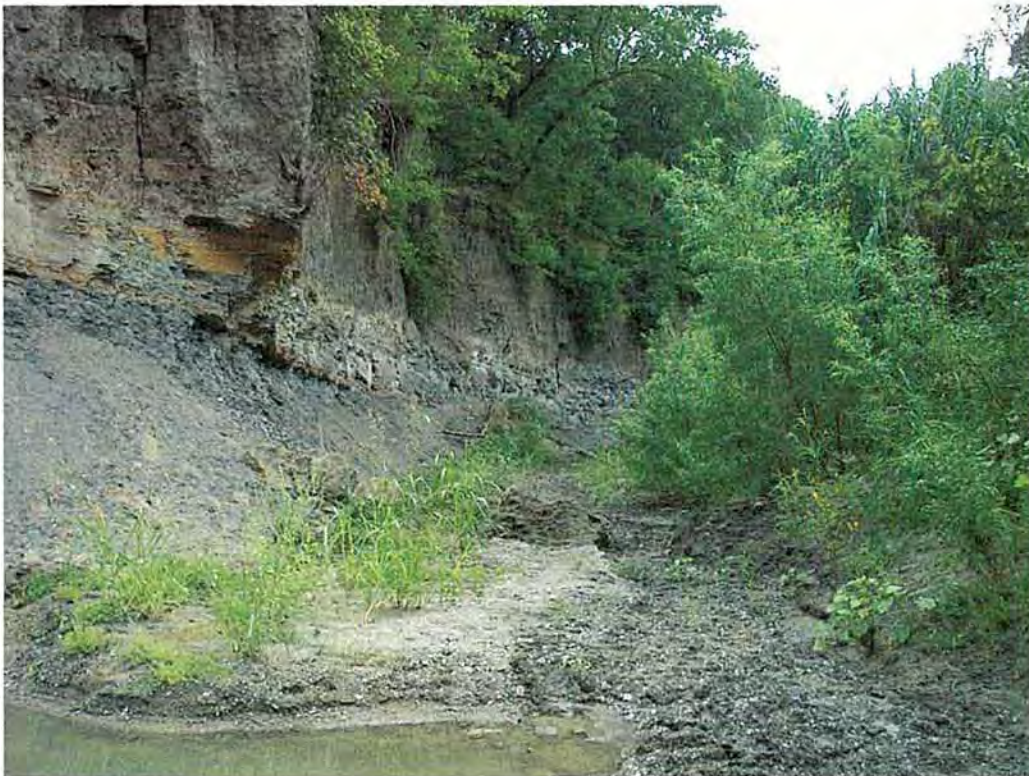
P15. Looking along shear vertical side slopes for one of the tributaries located along the North Sulphur River. This photograph was taken at the confluence with the North Sulphur River.
