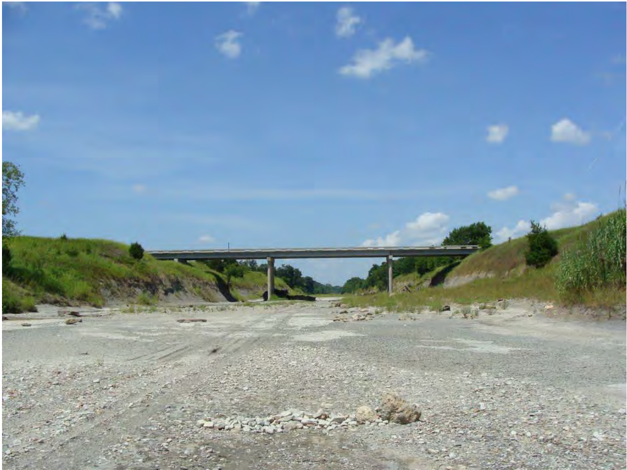
Figure 1. Photo of the North Sulphur River channel at the State Highway 34 bridge
