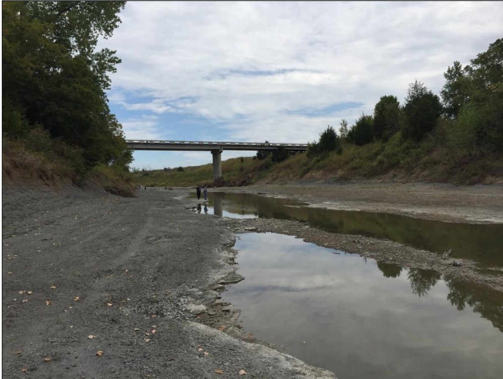
Photo 3-11: North Sulphur River pools at the existing SH 34 Bridge.
