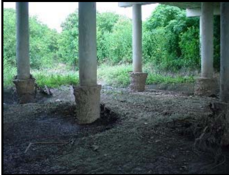
Culebra Creek - Culebra St Bridge Piers Scouring
