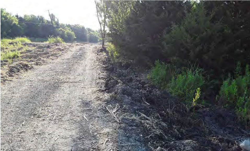
Photo 5: Construction disrupting connection of S-1 to the unnamed tributary.
