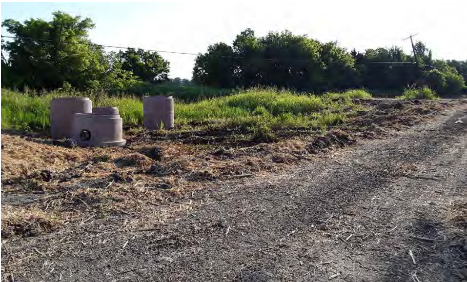
Photo 6: Construction disrupting connection of S-1 to the unnamed tributary.
