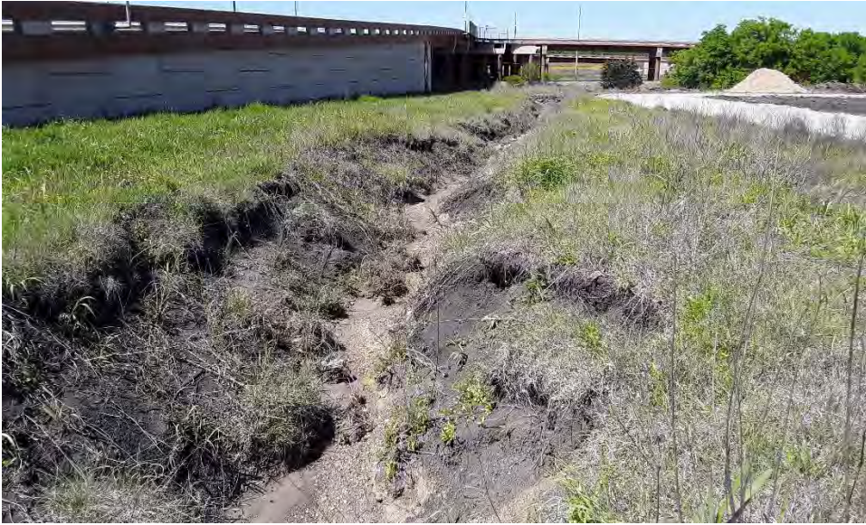
Photo 5: ED-1 - Man Made Drainage
