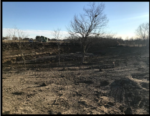
Photo 9 - View of Pond-1 during removal of silt. See Photo Location Map for location.
