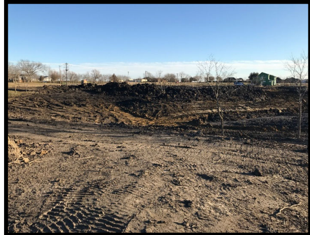
Photo 8 - View of Pond-1 during removal of silt. See Photo Location Map.
