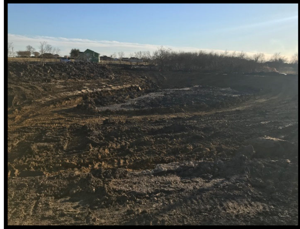
Photo 10 - View of Pond-1 during removal of silt. See Photo Location Map.
