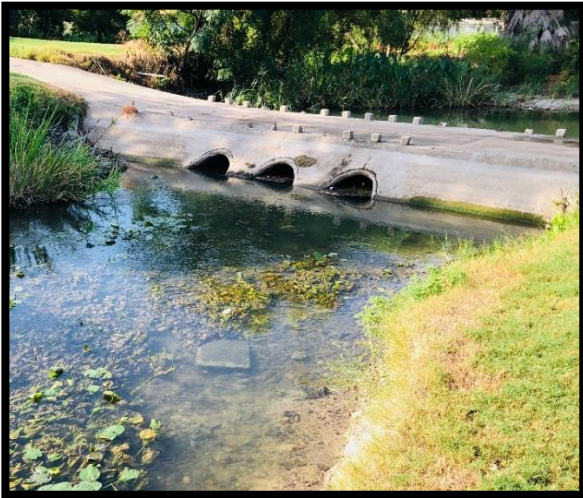
Figure 6. Low Water Crossing 3
