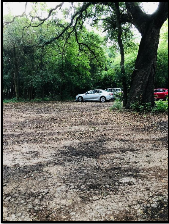
Figure 10. Severely Degraded Road/Non-Existent Habitat at the Avenue A Dead-End
