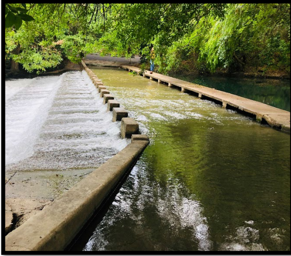
Figure 9. Low Water Crossing 1
