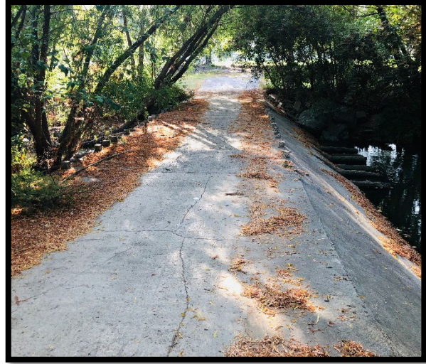
Figure 10. Low Water Crossing 2
