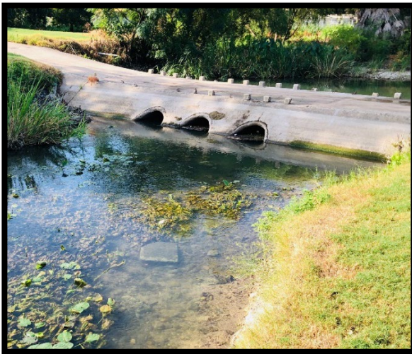
Figure 11. Low Water Crossing 3
