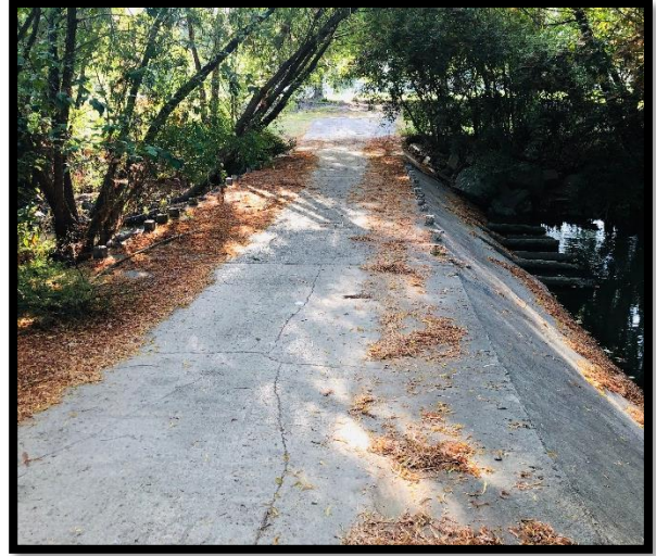
Figure 2-4. Low Water Crossing 2
