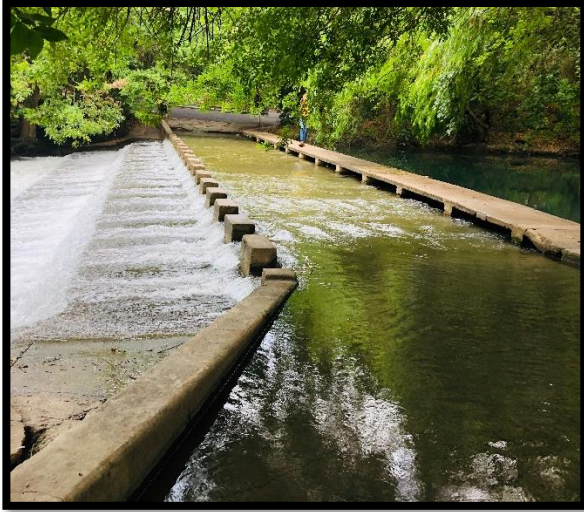
Figure 2-3. Low Water Crossing 1
