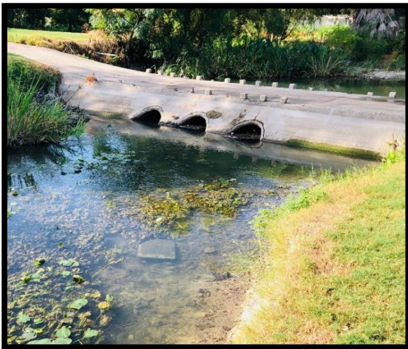
Figure 2-5. Low Water Crossing 3
