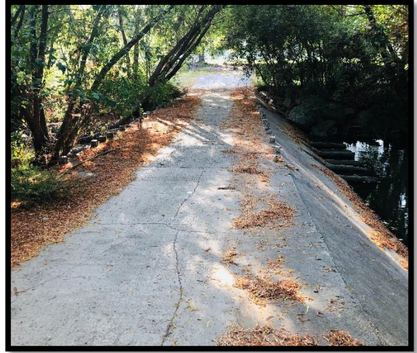
Figure 5. Low Water Crossing 2
