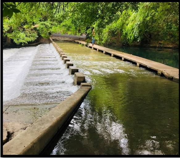
Figure 4. Low Water Crossing 1
