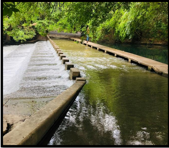
Figure 2-3. Low Water Crossing 1
