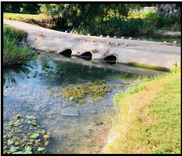
Figure 2-5. Low Water Crossing 3
