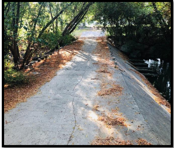
Figure 2-4. Low Water Crossing 2
