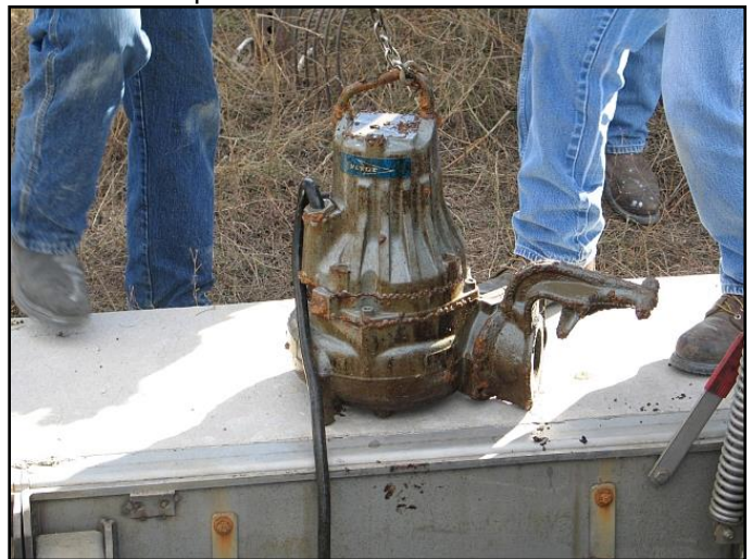
Figure 2. Water is supplied to Cell D by the pump pictured above, and to Cells E and E-West by a larger pump installed in a nearby vault.
