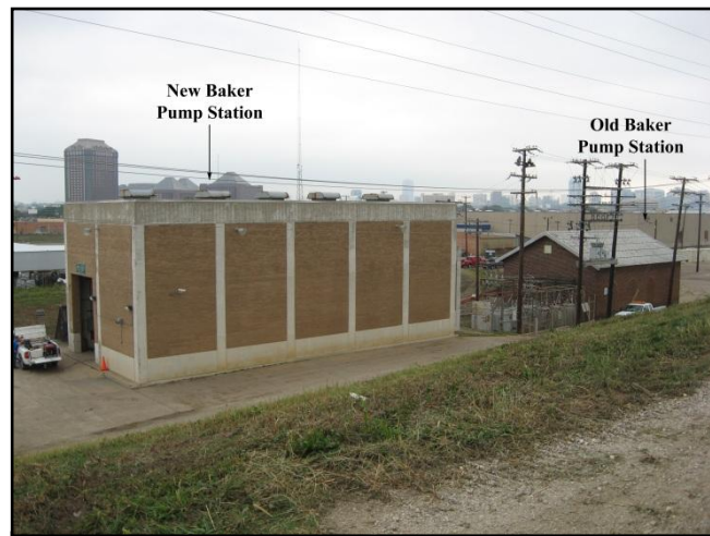
Figure 3-3 Baker Pumping Plant
