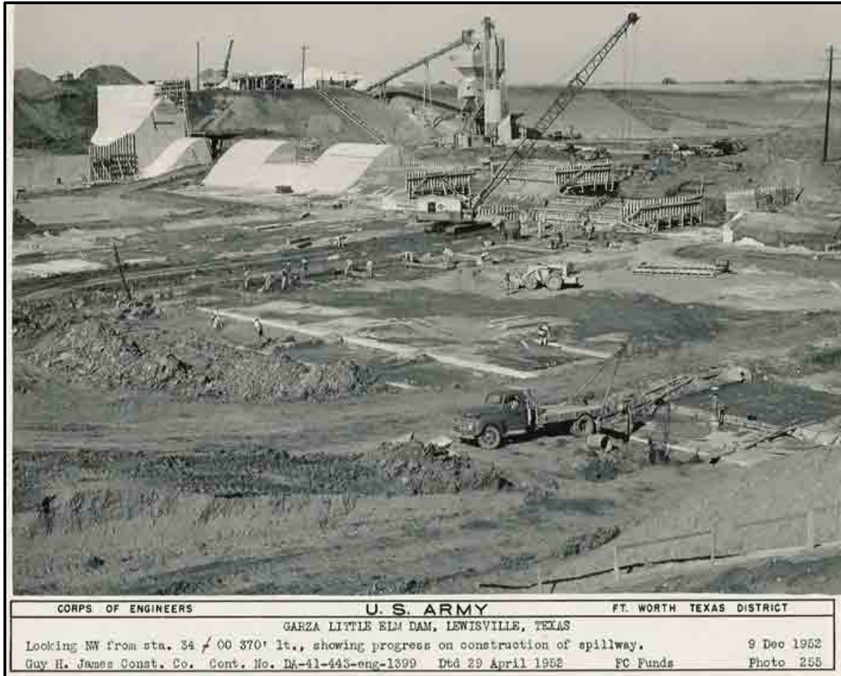
Figure 1.3 Construction of Lewisville Dam Spillway, 9 Dec 1952
