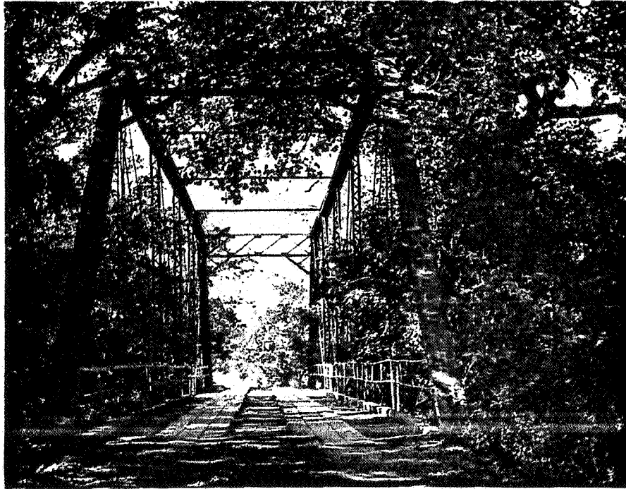
Figure 3. Willis Creek Bridge
