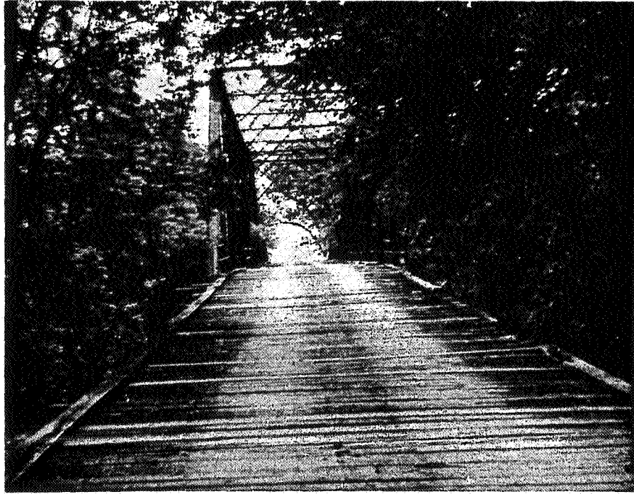
Figure 5. Approach Hoxie Bridge
