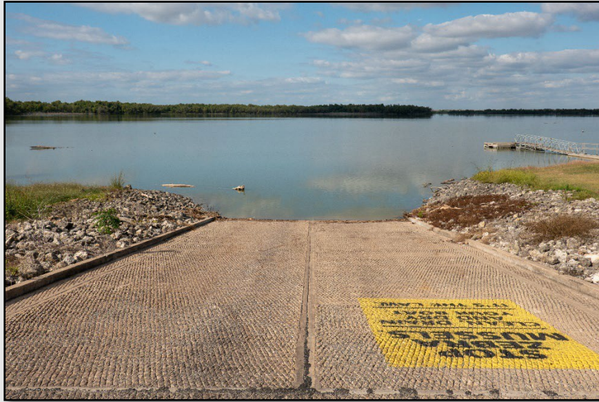
Photo 5-5 Willis Creek Park boat ramp
