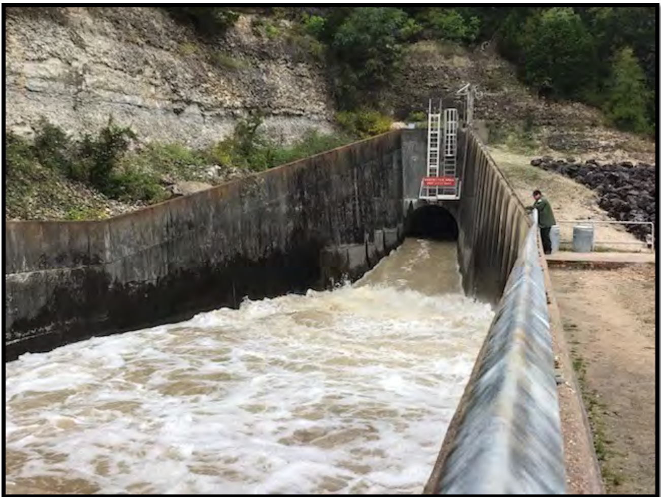
Photo 2-1 Downstream View of Outlet Works and Stilling Basin (Source: USACE Photo)
