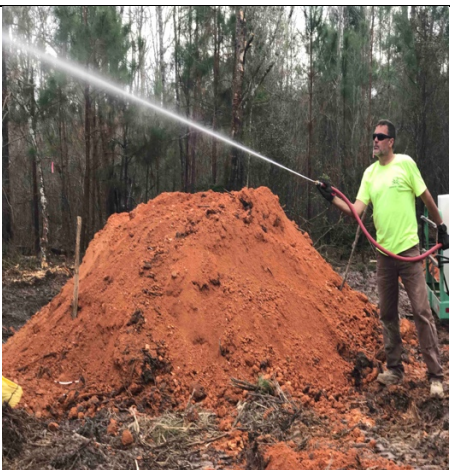
Area being wet down
