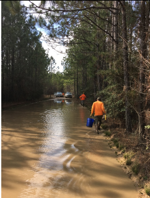
Standing water on roadway
