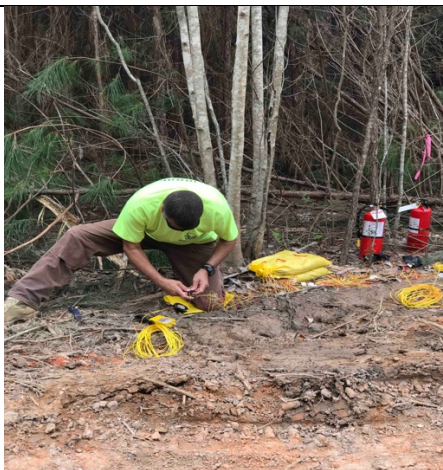
Electric detonator build up
