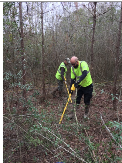
Mag and dig intrusive operations G-06
