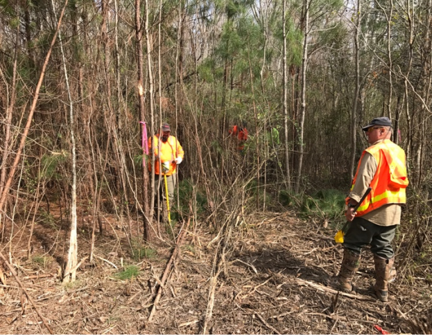
Clearing 30' buffer area around disposal location
