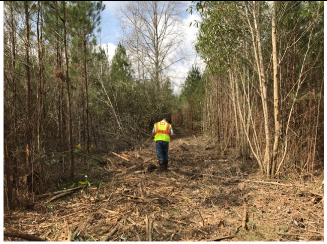
Cleared access path to disposal location
