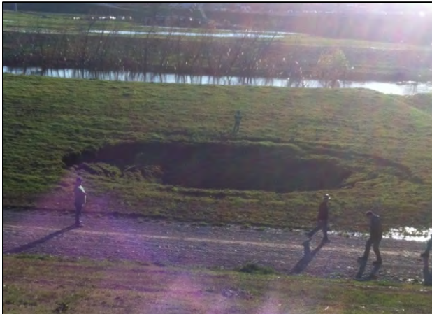
Figure 19 - Photo of the Sinkhole
