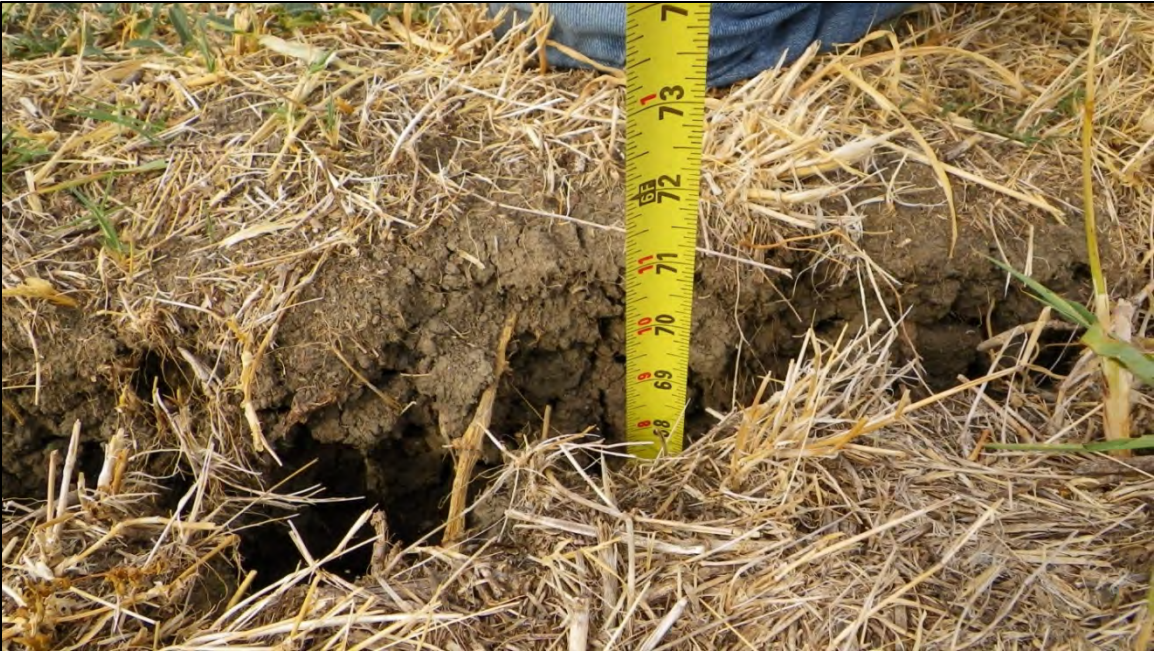
Depth of longitudinal cracking in the crest of the embankment.
