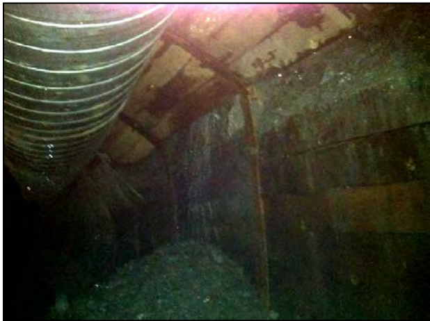
Figure 17 - Photo of the Initial Collapse
