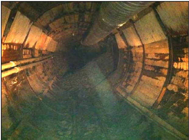
Figure 18 - Photo of the Collapse Progressing
