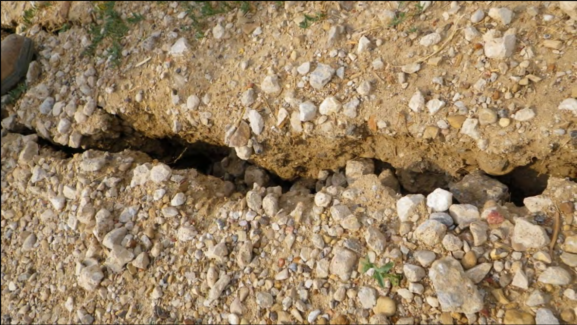
Longitudinal cracking in the crest of the embankment.
