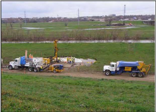
Figure 20 - Photo of the Remedial Grouting
