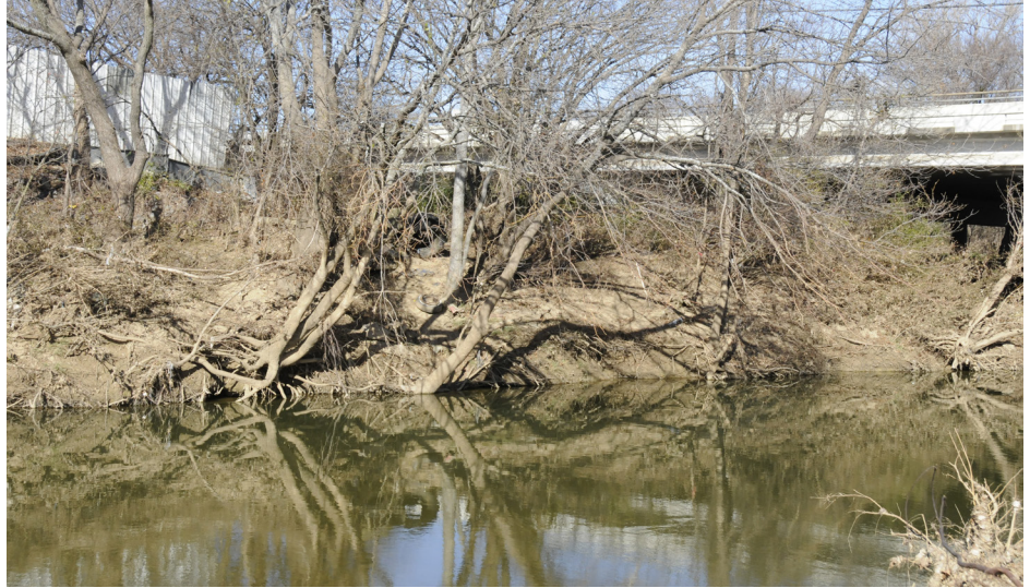
Kennedale Parkway, which has been closed by flooding, crosses Village Creek. Removing landfills in the floodway on both sides of the creek here are among the alternatives a feasibility study would examine.
