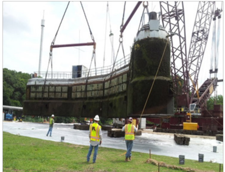
Workers remove the Submarine Theater from the long-closed Aquarena Center.
