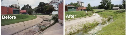
capacity was only 25 percent of the 100-year peak runoff. The project tripled flow capacity by widening the channel bottom to 30 feet along a 7,860-foot stretch of Pecan Creek. Grass-lined banks had
