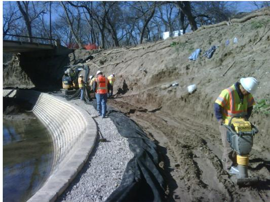
was not stabilized, the stream banks would continue to fail. At the current rate of erosion, both the embankment and the bridge were likely to be negatively impacted within the next five years. The site is adjacent to a Dallas County park.
