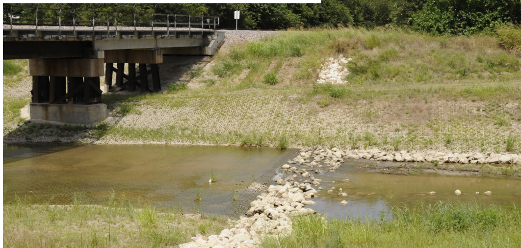
Continuous articulated concrete was placed down one bank, across the creek bottom, up the other side on this reach. Two years later, it had a more natural look.
