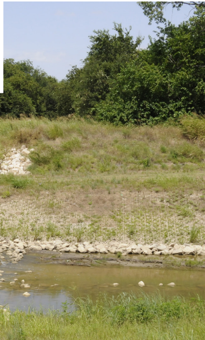
Continuous articulated concrete was placed down one bank, across the creek bottom, up the other side on this reach. Two years later, it had a more natural look.
