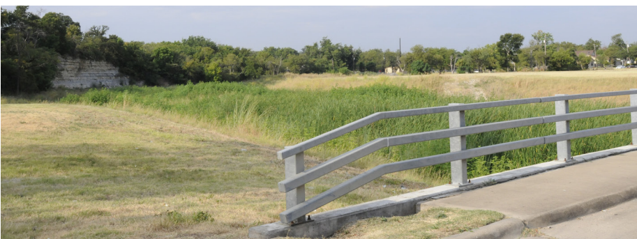
The widened channel seen from the White Settlement Road Bridge.
