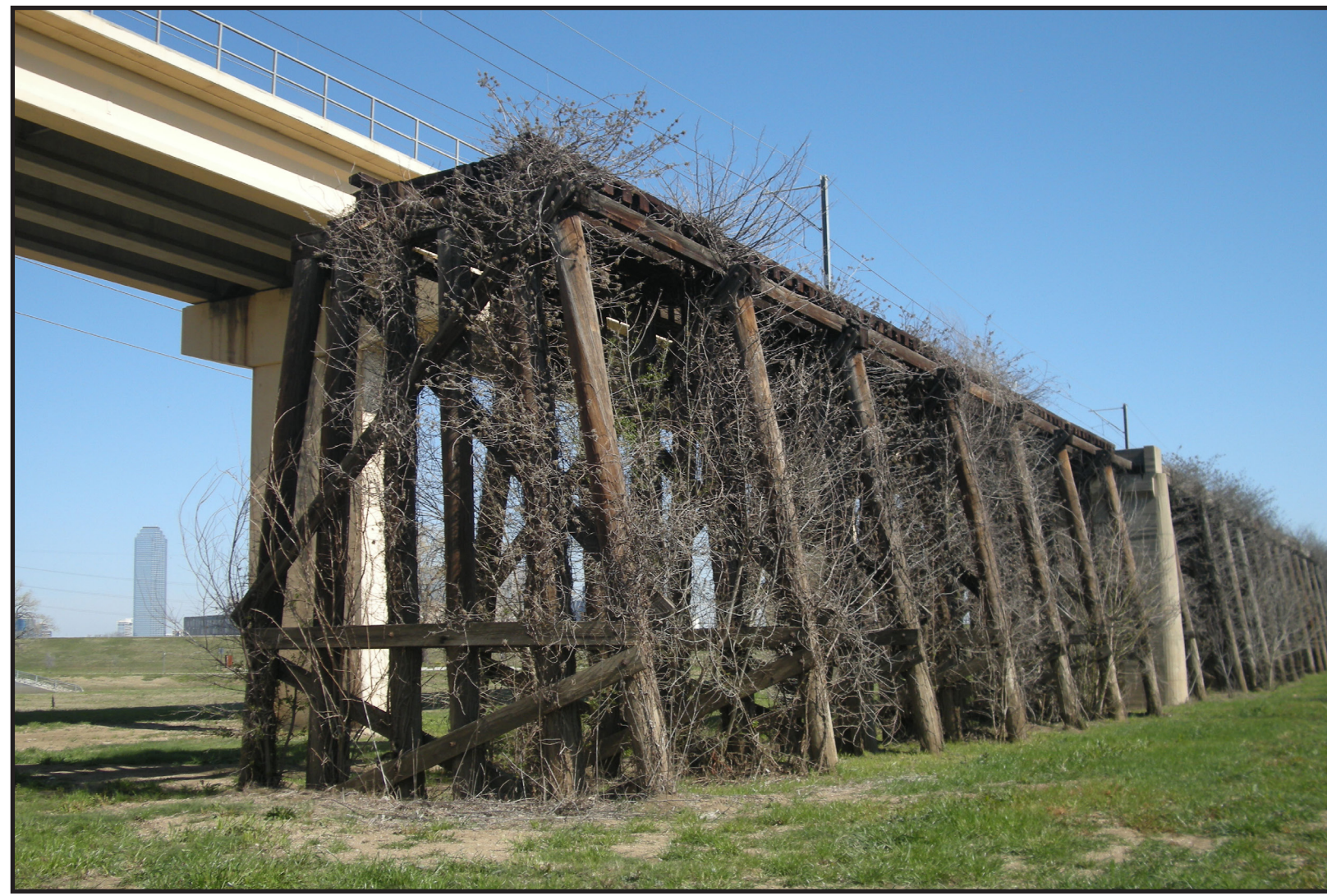
Existing Wooden Trestle (to be removed)
