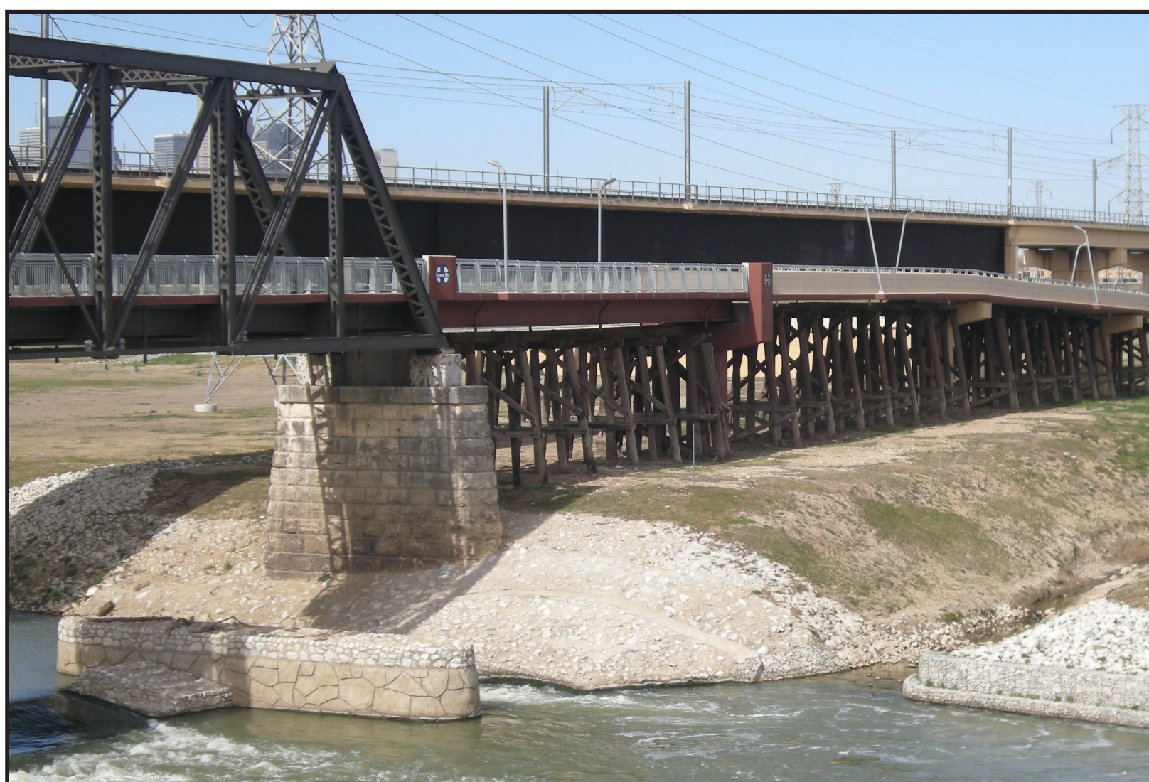
Existing AT&SF Open Steel Truss Center (to remain) and Santa Fe Trestle Trail
