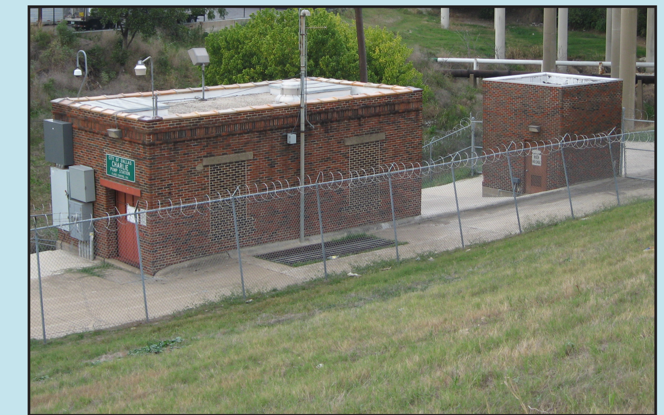
Charlie Pump Station
