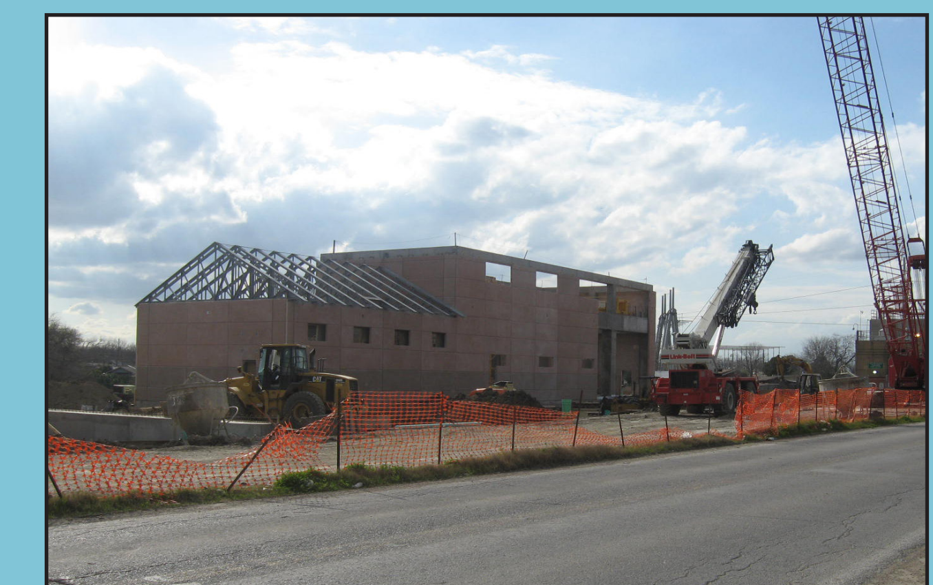
Construction at the Pavaho Pump Station
