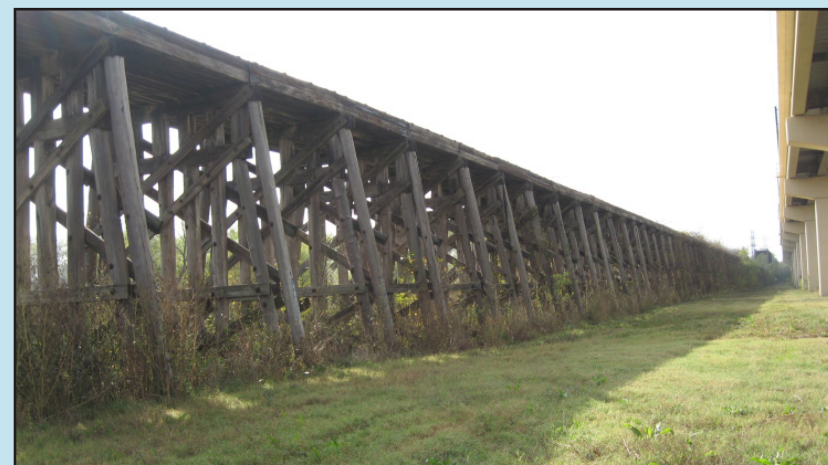
AT&SF Railroad Bridge Wood Trestle
