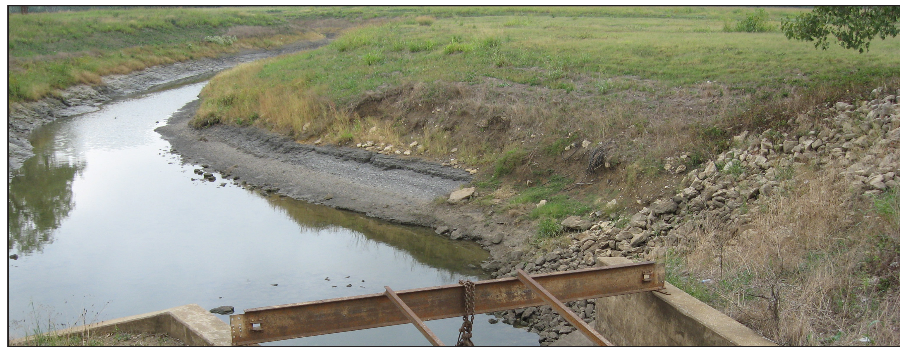
Hampton Pump Station Outfall
