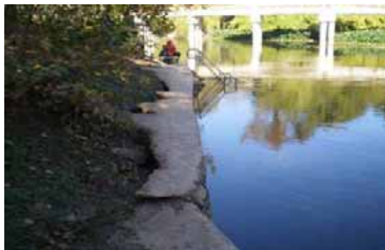
Photograph 4-3. Concrete Headwall Proposed for Removal
