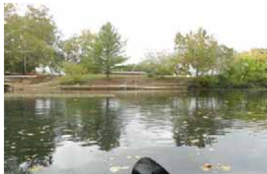
Photograph 4-4. Concrete Headwall Proposed for Removal
