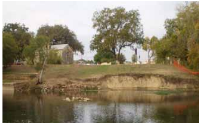
20 21 Photograph 4-2. Area of Degraded Shoreline Where 22 SHORE1 Is Proposed
