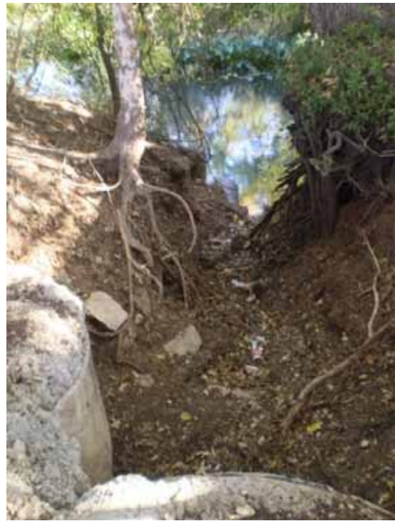
Photograph 4-5. Example of Existing Drain Requiring Improvement
