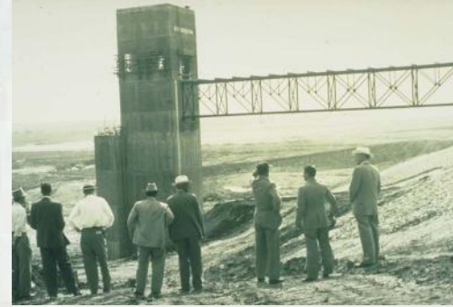
Benbrook Dam Construction 1950
