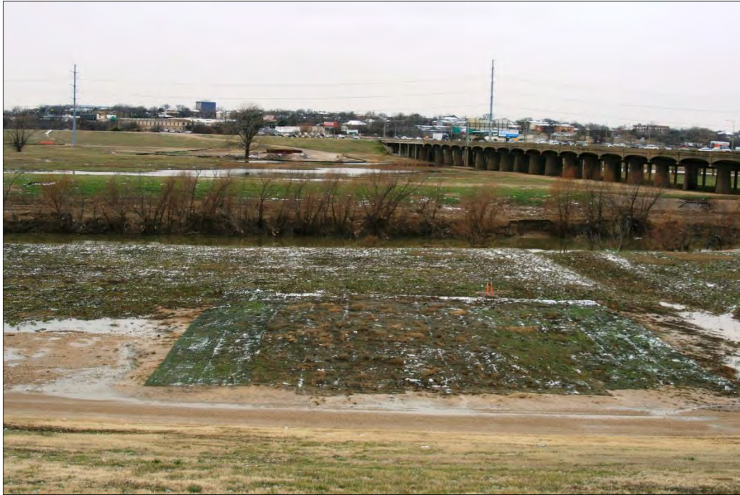
Photo 7: View of the project alignment from on top of the East levee, looking southwest. The revegetated rectangle in the center of the photo is the filled depression.
