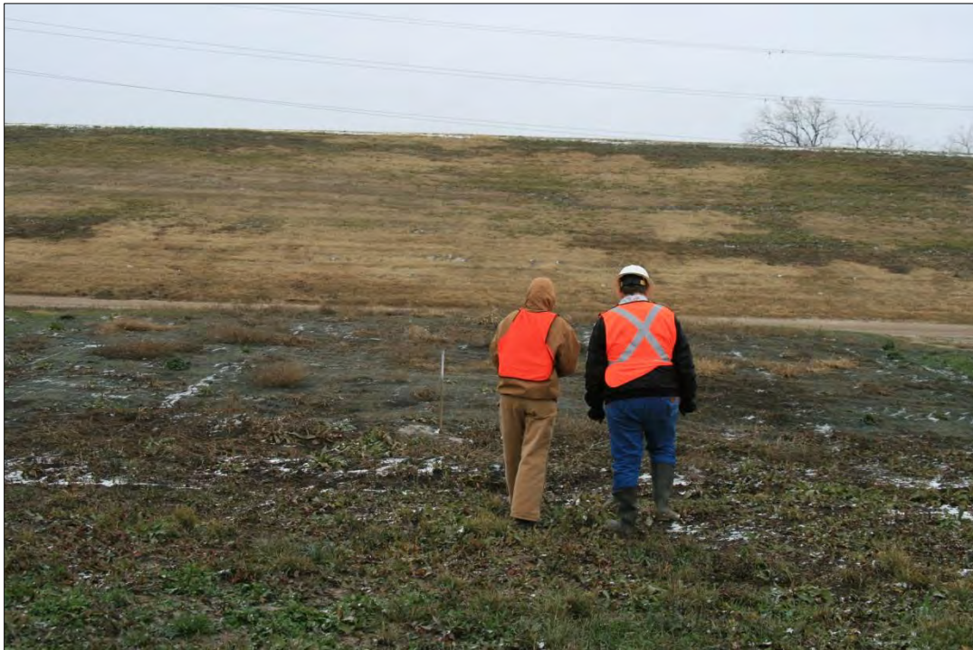
Photo 6: View of East levee from the project alignment, looking northeast. Depression area (discolored) appears in the center of the photograph.
