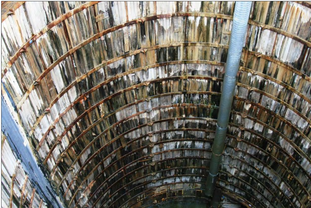
Photo 10: View looking inside the access shaft (already constructed as part of development of the first tunnel).
