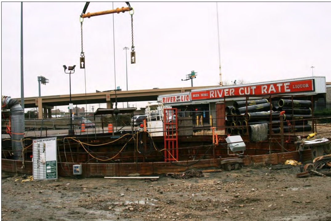
Photo 2: Access shaft at the Cadiz Street Pump Station, looking south.
