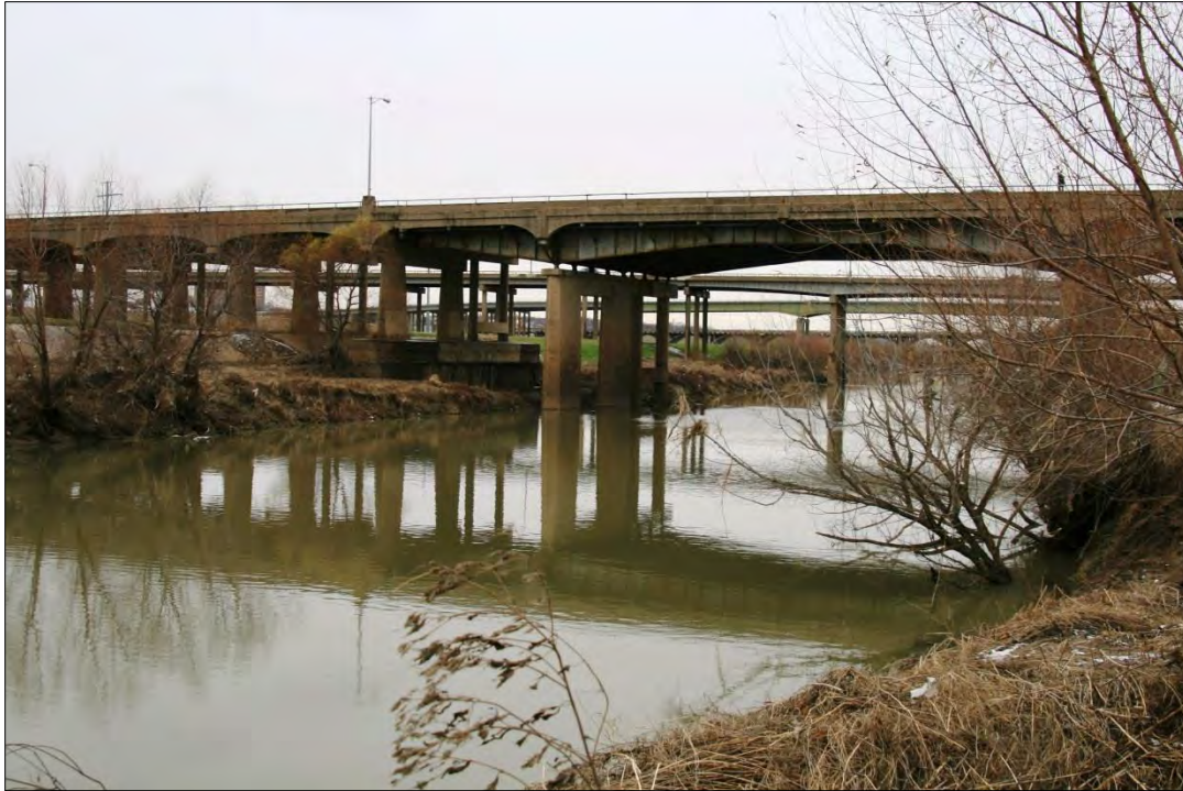
Photo 5: I-35 North / Cadiz Street crossing the Trinity River, looking north.
