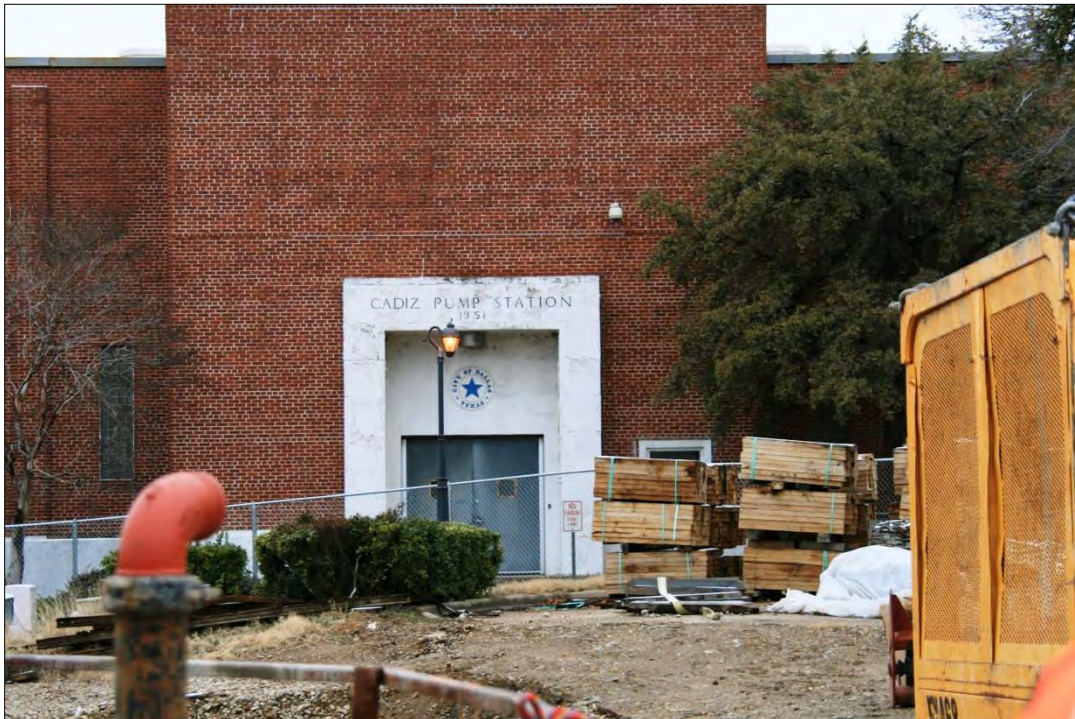
Photo 4: Cadiz Pump Station and construction staging surrounding the access shaft (looking northwest).
