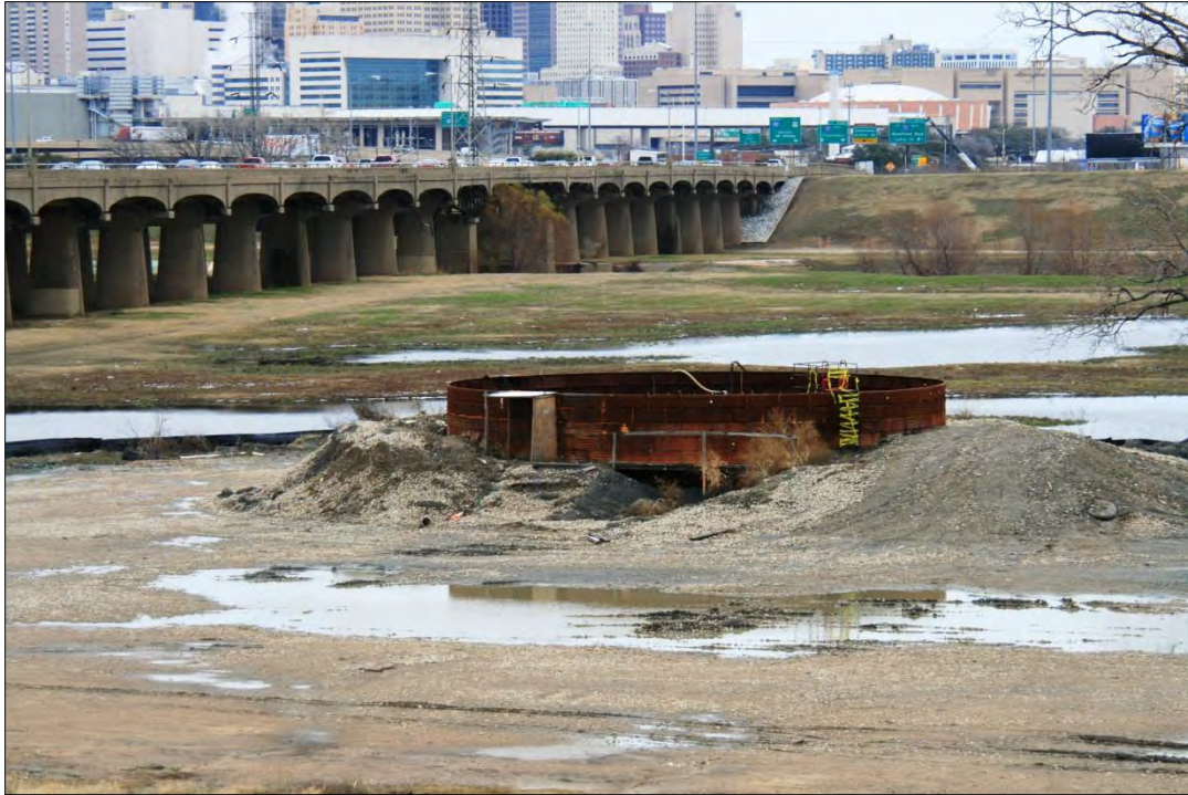
Photo 1: Access shaft to the southwest of the Trinity River, looking north. Construction has already been approved and work commenced for the first tunnel.
