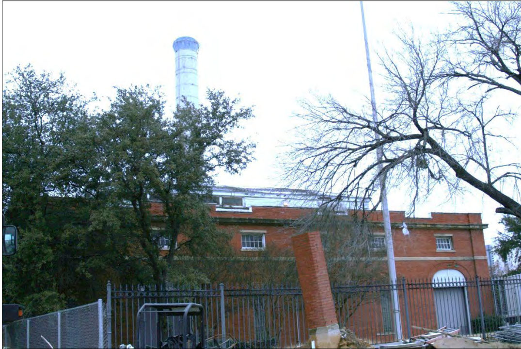
Photo 3: Original Cadiz Pump Station adjacent to the construction of the access shaft (looking north).
