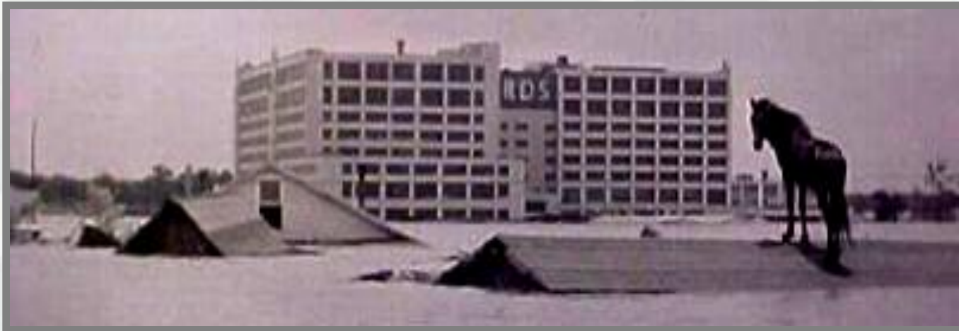
Montgomery Ward building, 1949 Fort Worth flood
