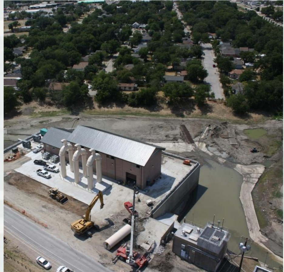
2012 New Pavaho Pump Station
