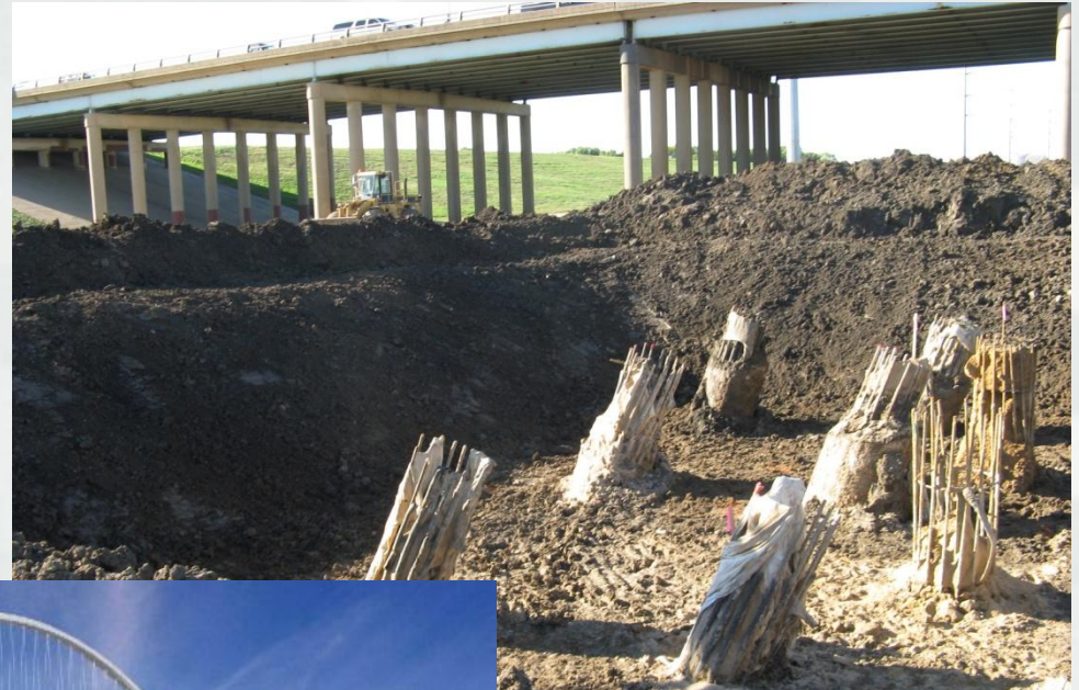
New drill shafts for I-30 Margaret McDermott Bridge
