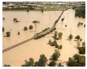
Modification of the abandoned AT&SF Bridge on the Trinity River, shown above during a 1989 flood. The bridge collects storm debris in its piers which, like a stopper, cause floodwaters to back up into the system. The modification includes removal of earthen embankments and most of the piers. The historic Santa Fe Trestle, the new Santa Fe Trestle Trail and some of the historic wooden piers protected by the trail will be preserved.
