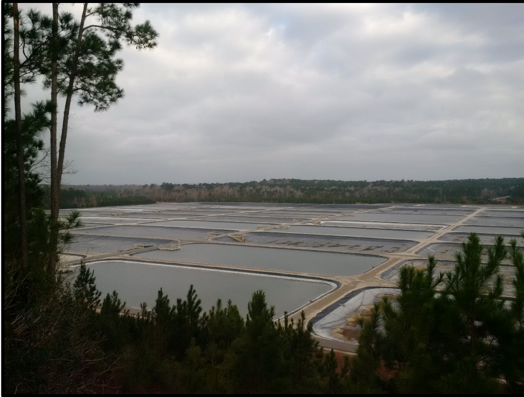
1034 1035 Photo 2-1 John D. Parker East Texas State Fish Hatchery near Sam Rayburn Reservoir 1036 (USACE Photo)
