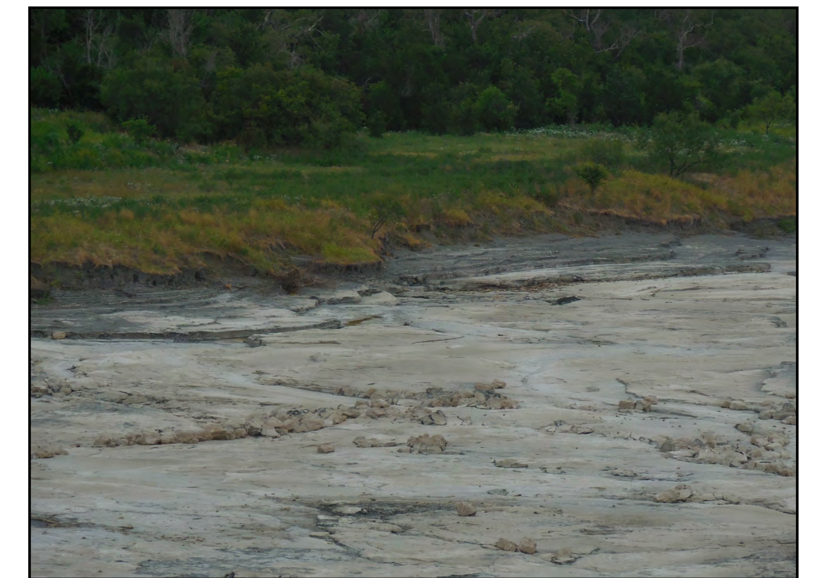
Scour Downstream of the Spillway Apron
