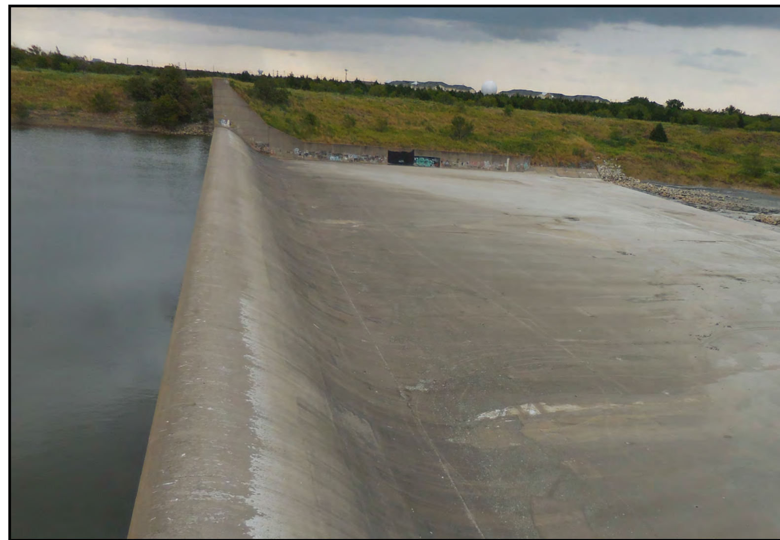
Spillway and Apron
