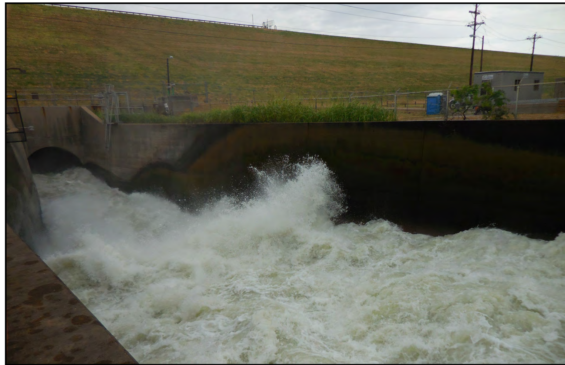
Lewisville Lake outlet conduit at full discharge.
