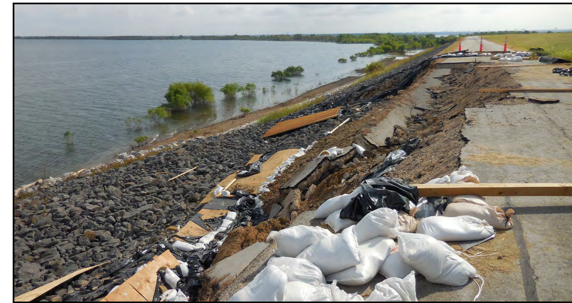
Ongoing repairs to a slide at Lewisville Lake resulting from the May 2015 storms.
