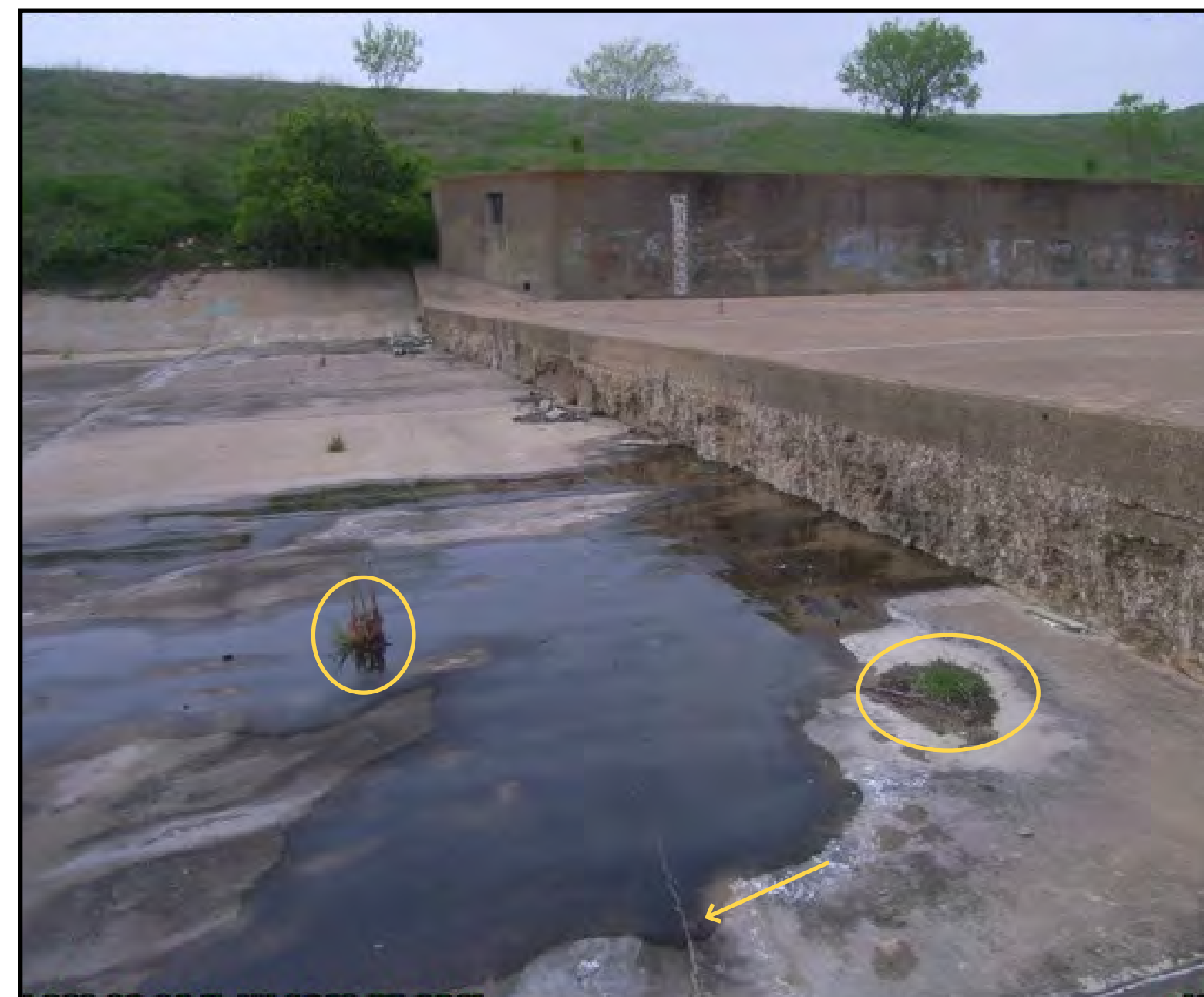
Cracks in the Spillway Apron
