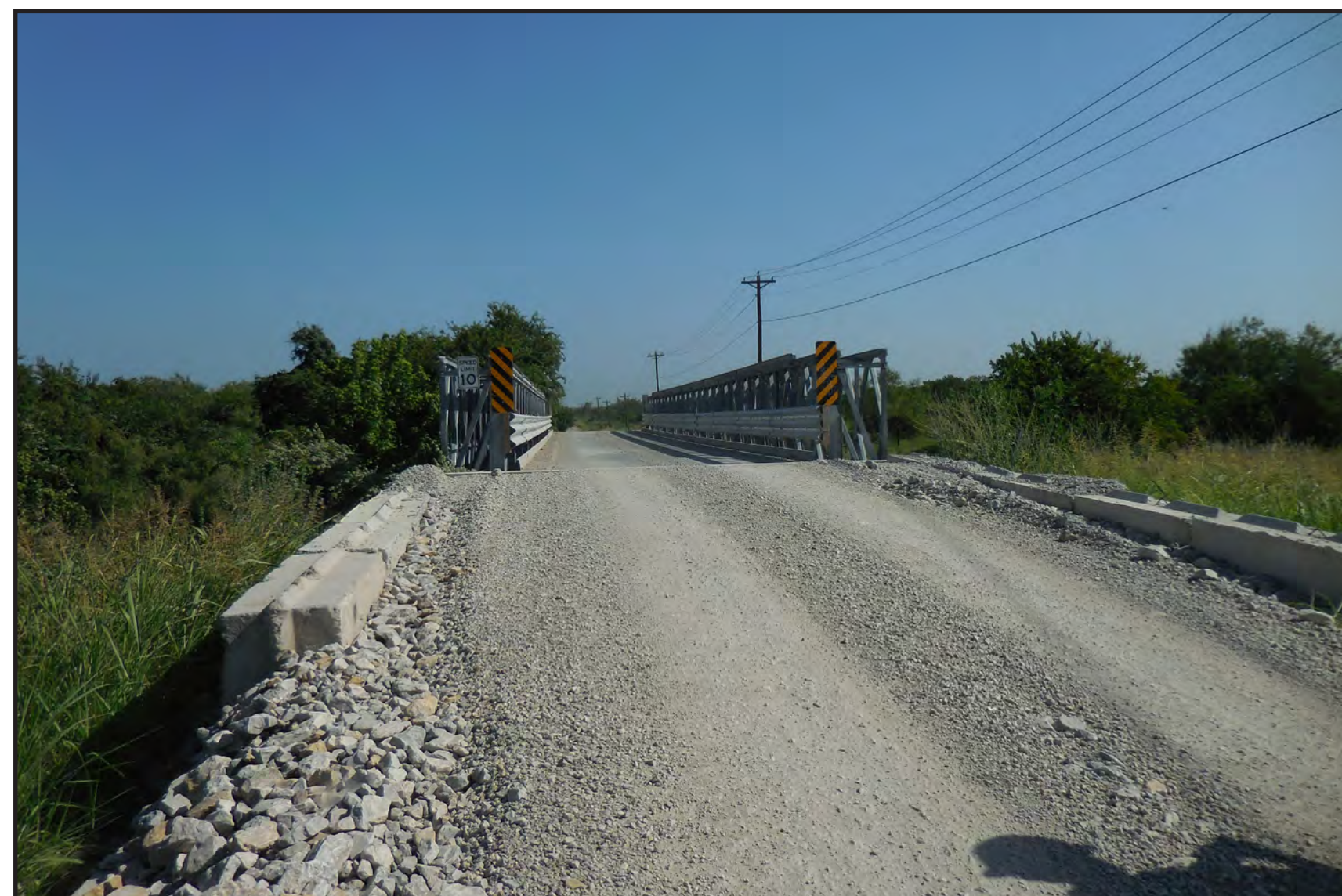
Existing temporary bridge superstructure serving Fish Hatchery Road over the Kansas City Southern Railroad. This bridge is scheduled to be removed by the end of 2016.
