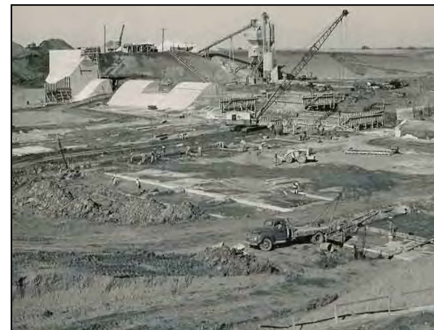
Construction of the Lewisville Dam (1952)
