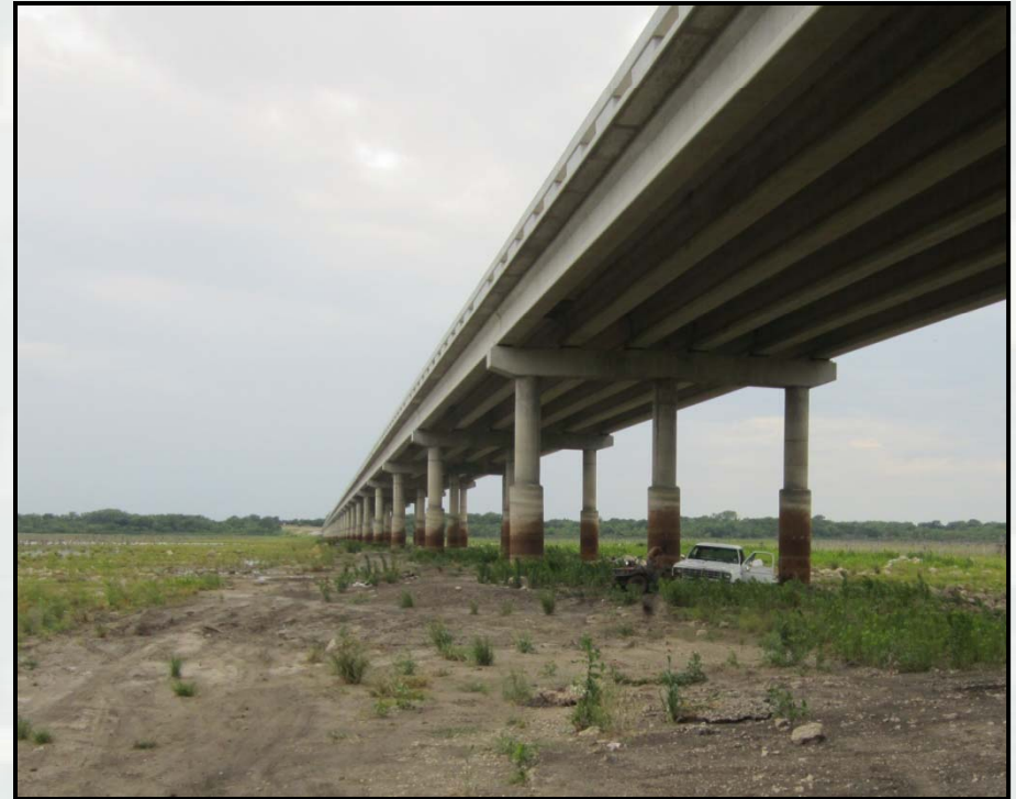
FM 3286 Bridge, Summer 2014
