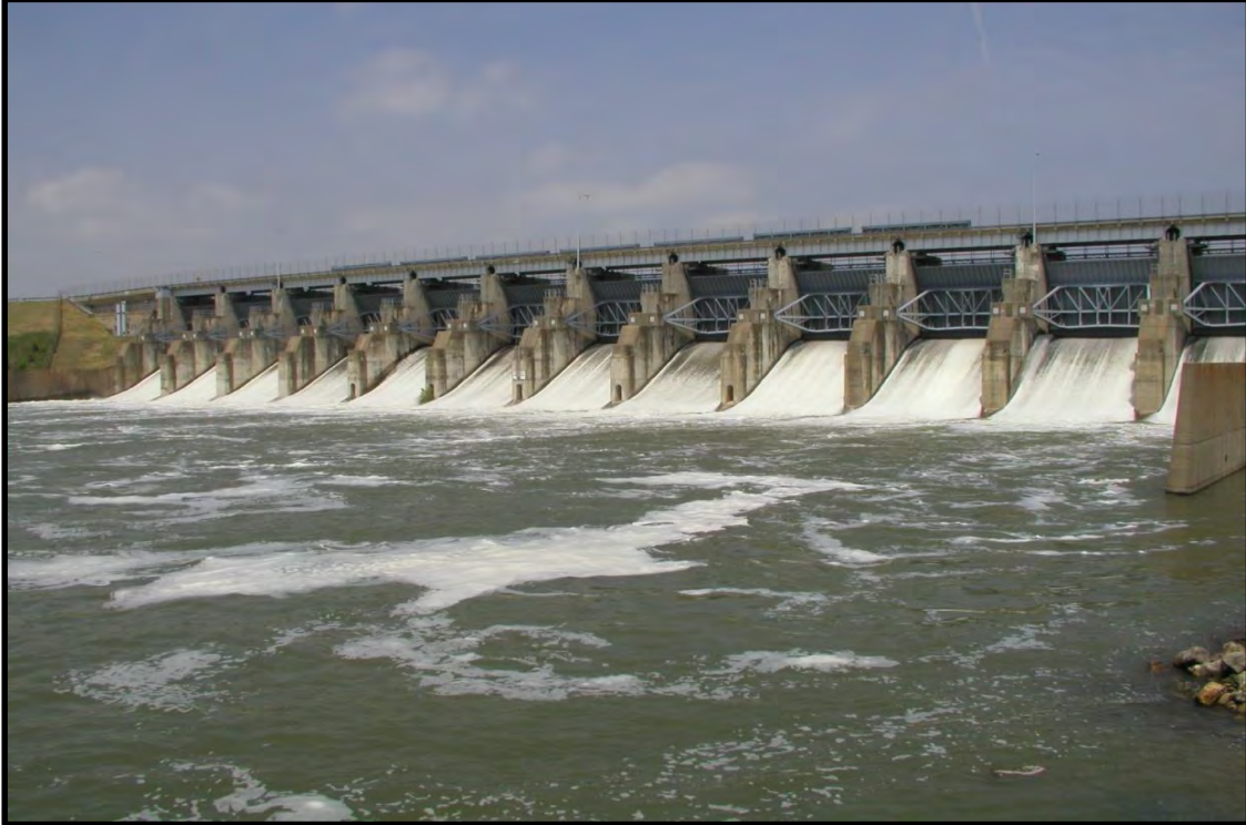
2269 2270 Photo 5.1 Lavon Dam Tainter Gates during a Major Release of Stored Floodwater 2271 (USACE photo)
