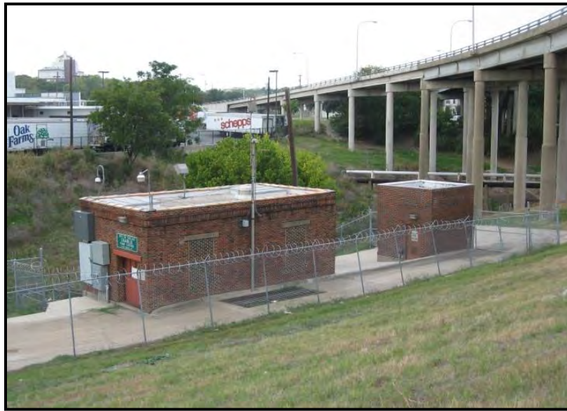
Photo 6: Charlie Pumping Plant
