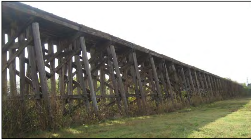
Figure 3.11-1 AT&SF Railroad Bridge Wood Trestle
