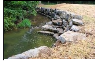
Channel bank armoring
