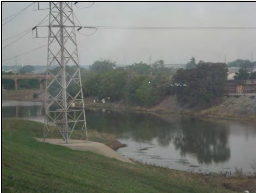
Photo 15: Able Sump; looking northeast
