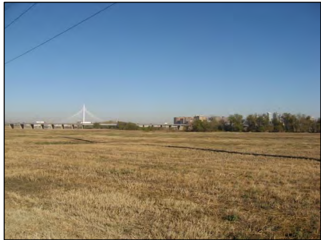
Photo 9: Existing conditions looking north on the west side of the Dallas Floodway with the Margaret Hunt Hill Bridge in the background
