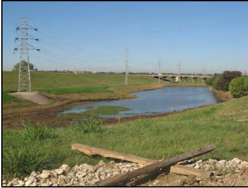
Photo 3: Grass-covered Levee (left) and Overhead Utilities
