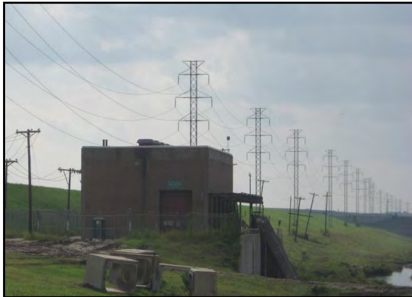
Photo 5: Hampton Pumping Plant
