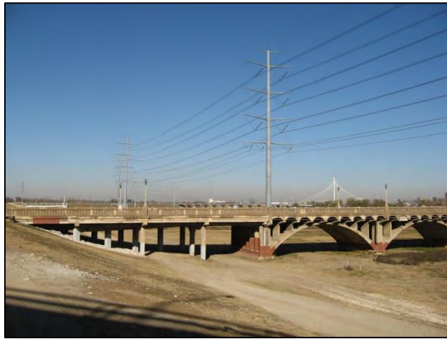
Photo 11: Existing conditions looking north on the west side of the Dallas Floodway with the Margaret Hunt Hill Bridge in the background
