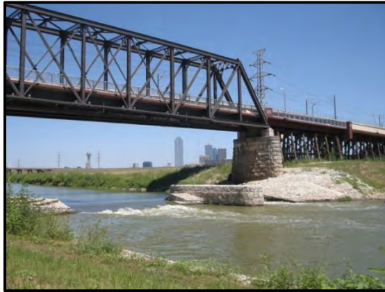
Photo 1: Existing AT&SF Railroad Bridge Steel Truss
