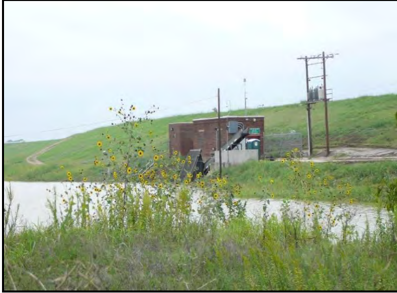
Photo 7: Delta Pumping Plant
