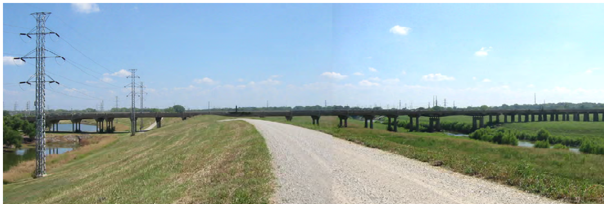
The structural approach to flood protection focuses on the levees. A view of the levee top today; an amazing place to be were it part of the public realm.
