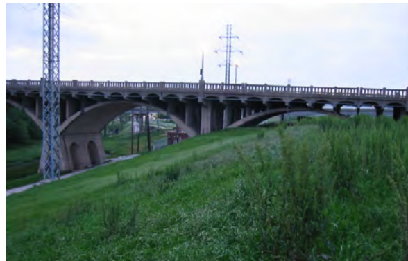
The Houston Street Viaduct.
