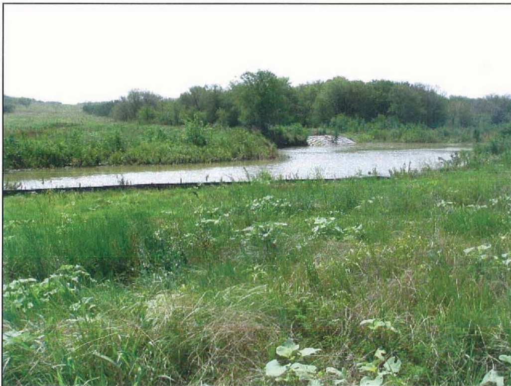
Figure 21: View of Tributary 10 (Soap Creek) looking downstream, facing southeast toward the crossing.
